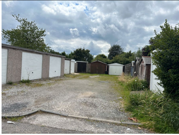
Church Avenue, looking south.
