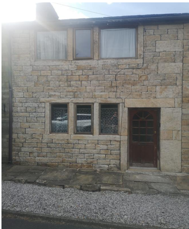
Front Elevation of No.8 Paul Row
