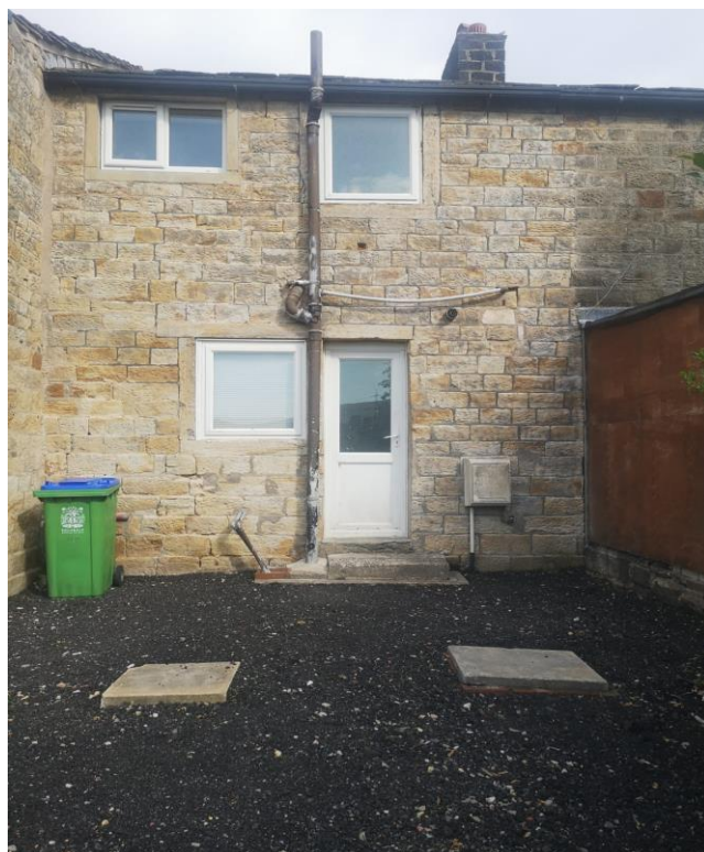
Rear Elevation of No.8 Row
