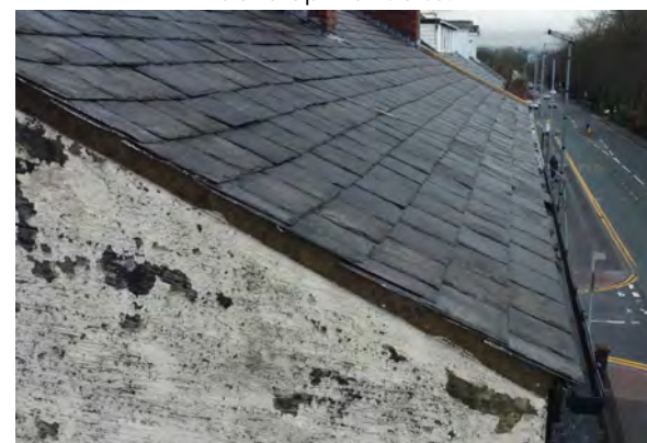
Photo 7 - Building to the east of the development site, older style and slate covered.
