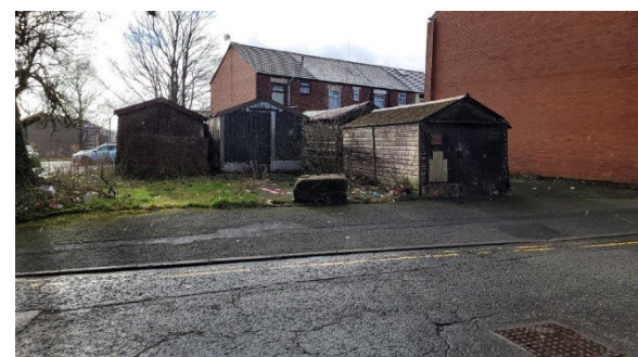
Block B – Existing Garages from the North
