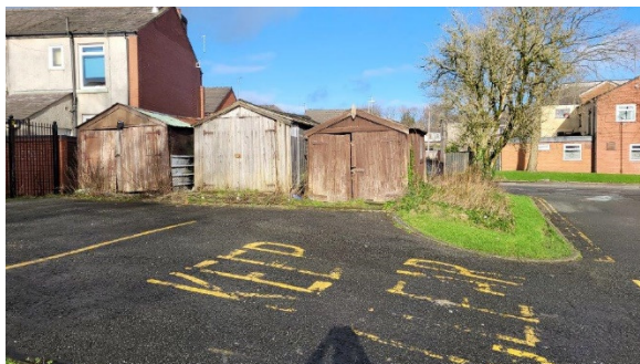
Block B – Existing Garages from the South
