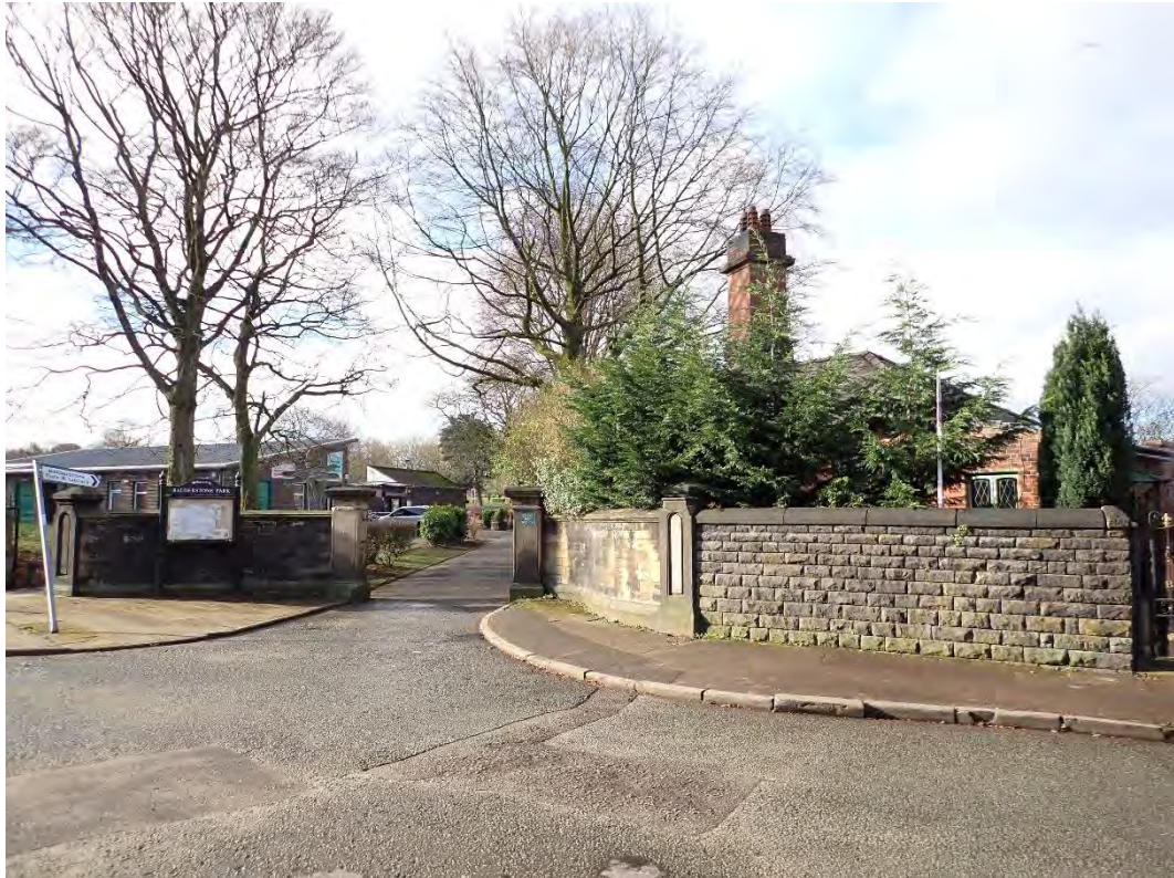
Photograph 5: Entrance to Balderstone Library and Park. Formerly the entrance to Balderstone Hall, constructed in the 19th century together with the lodge (705.1.1)
