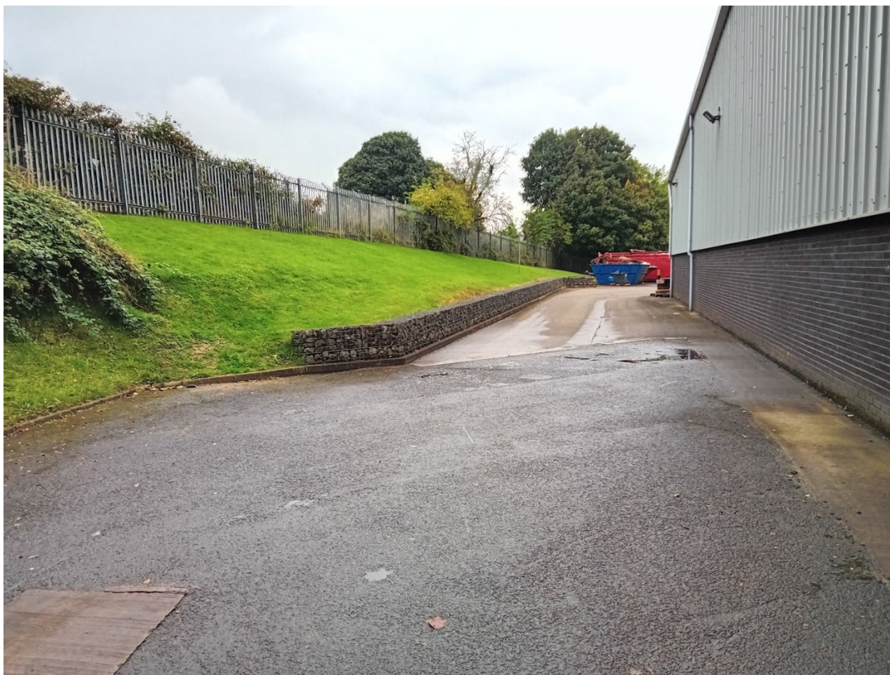
Photograph of access road to northwest of garage building. Note embankment with railway beyond to the left and service scars on road surface. Taken looking northeast.
