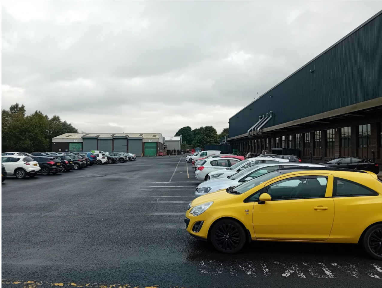
Photograph of carparking area showing main building (right) and smaller garage building (left). Taken looking northwest.
