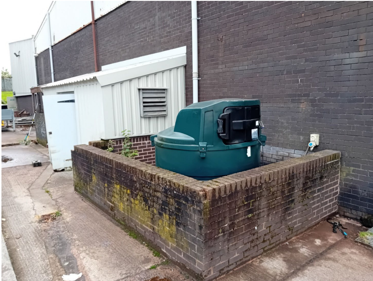
Photograph of above ground storage tank near southwest corner of garage building. Taken looking north.
