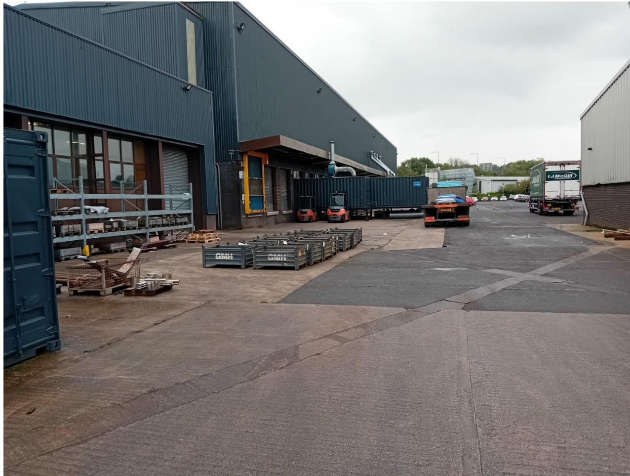
Photograph of storage areas to the west of the main building. Note service scars on road surface. Taken looking southeast.
