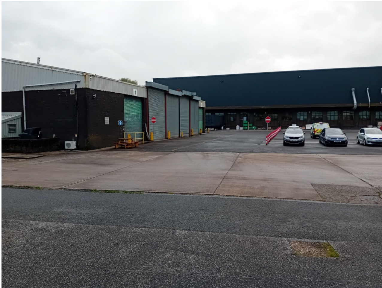
Photograph with garage building in the foreground and the main building in the background. Taken looking northeast.
