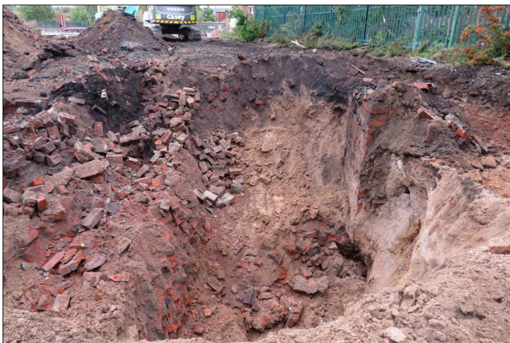
Plate 7: Excavated area following removal of chimney base 206 , depth in excess of 3m (no scale)
