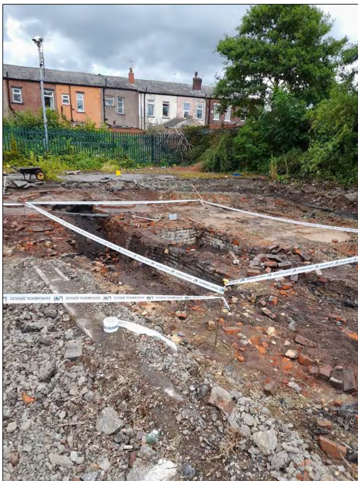
Plate 6: Areas of asbestos contamination in Trench 2
