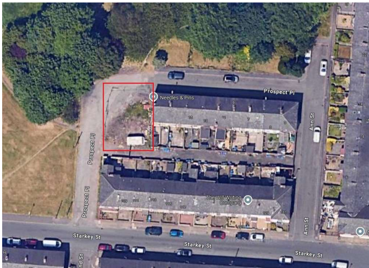
Aerial view of existing site
