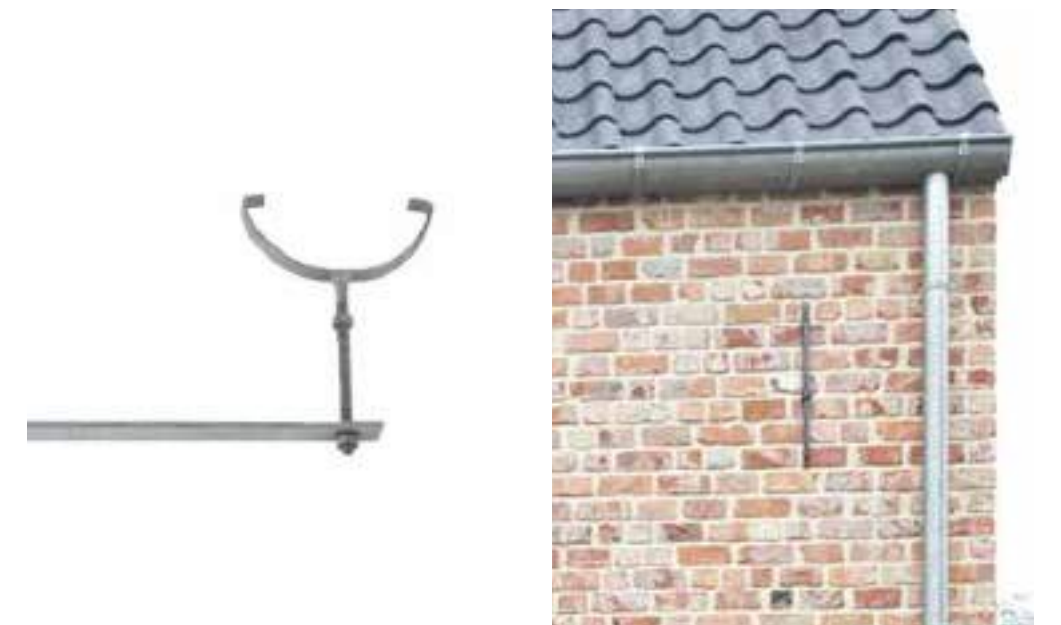
Gutters and Downpipes - half-round galvanised downpipes and gutters on rise and fall brackets
