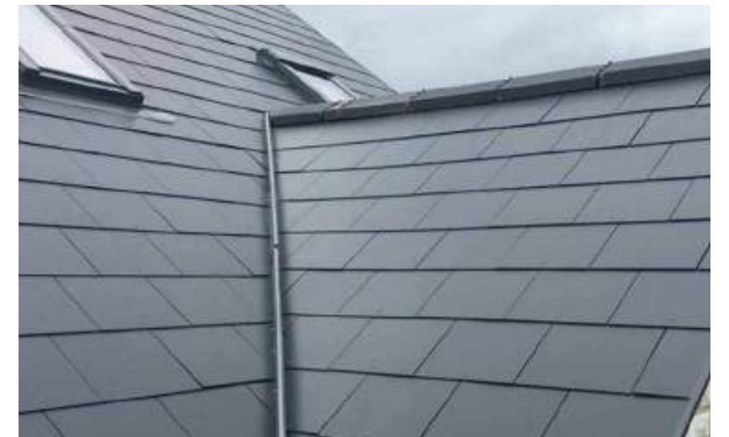
Fibre Cement Roof Tiles to houses
