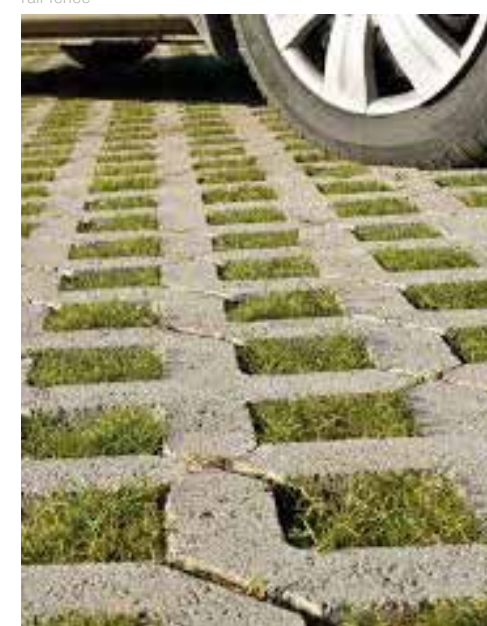
Parking within grassed areas - Tobermore Turfstone grass paving system
