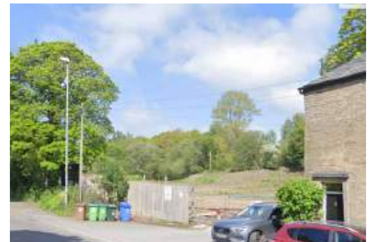
ENTRANCE TO SITE - BURY &amp; ROCHDALE OLD ROAD
