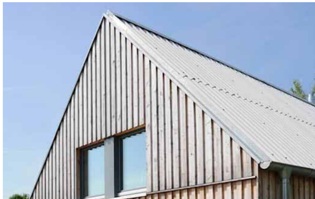
Sinusoidal Fibre Cement Roof on Commercial Unit
