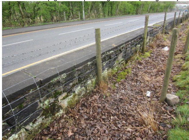
Photo 5: Stone wall at western site boundary with Hollingworth Road beyond
