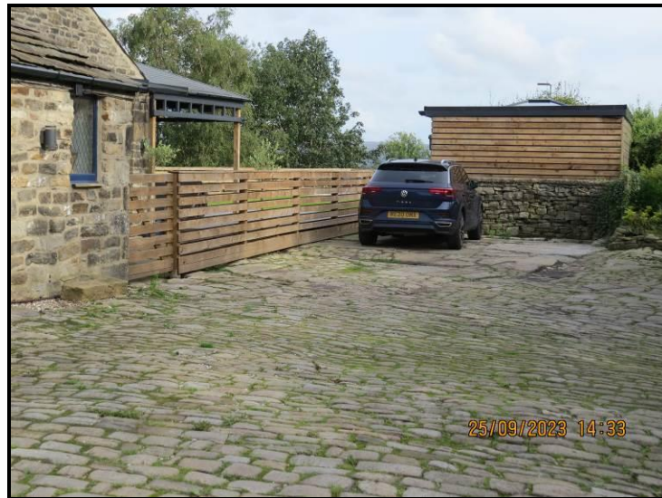
Photograph 002 Courtyard to South East elevation of Crossfield Barn
