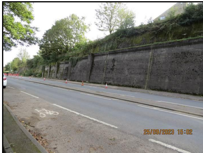
Photograph 011 Whitworth Road, retaining wall and upper slope
