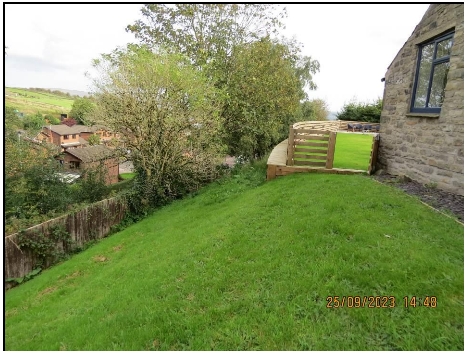
007 Gable to house and lower boundary fence
