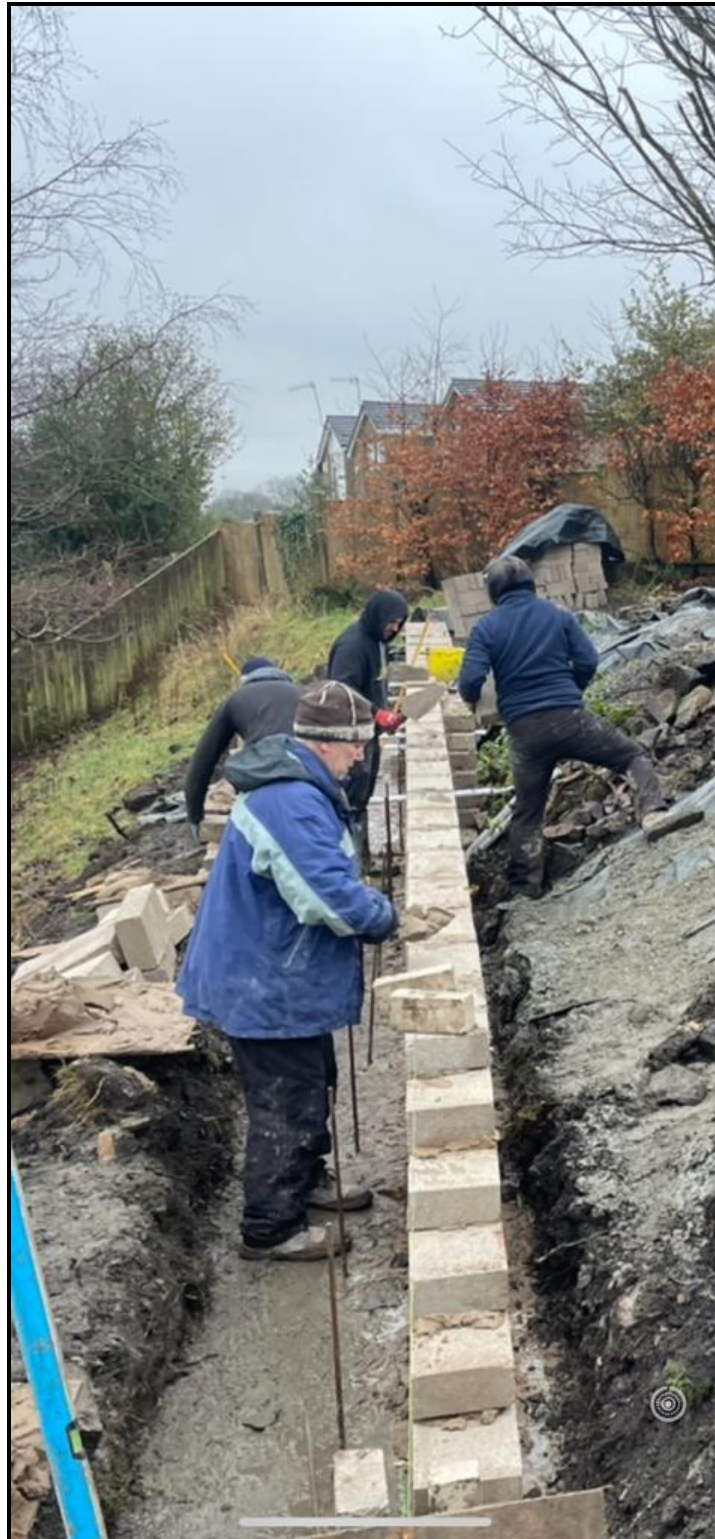
002E Inner leaf construction looking North West – South East
