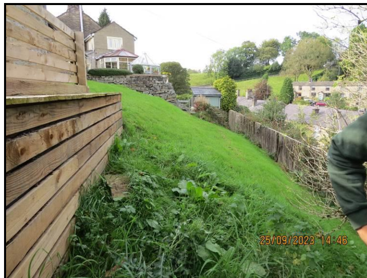
Photograph 006 Existing garden slope 29° looking South East – North West
