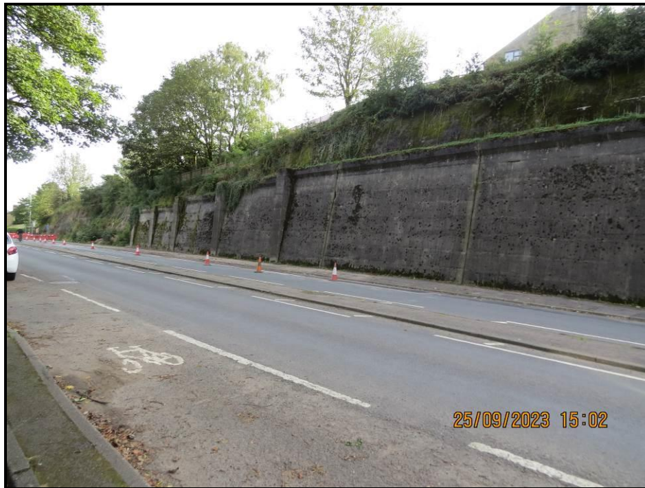
011 Whitworth Road, retaining wall and upper slope
