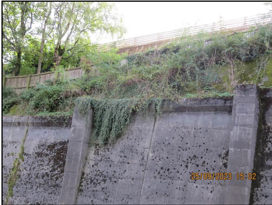
013 Close up of upper embankment
