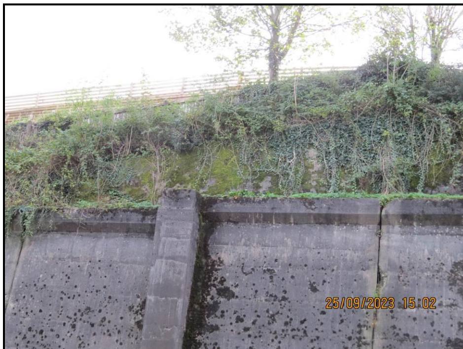
012 Close up of upper embankment
