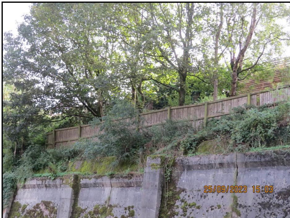
014 Lower timber boundary fence and existing foliage
