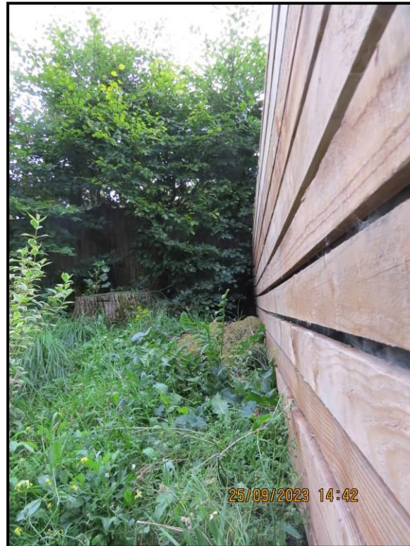
005 Return wall South East frontage
