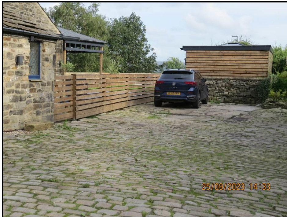
001 Courtyard to South East elevation of Crossfield Barn
