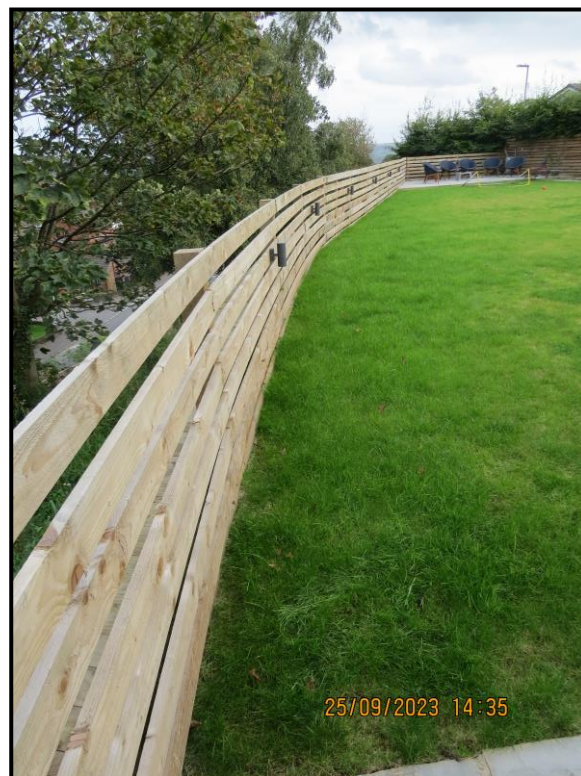
002 Wall profile looking North West – South East
