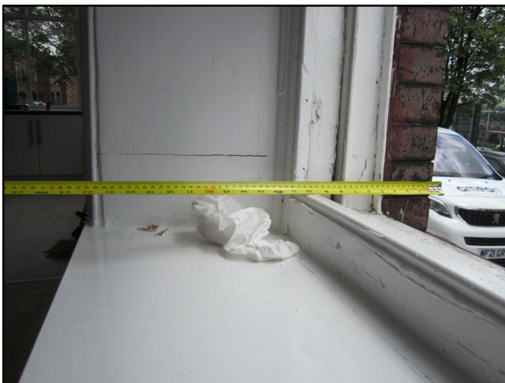
Photograph 6. External walls to the existing building
