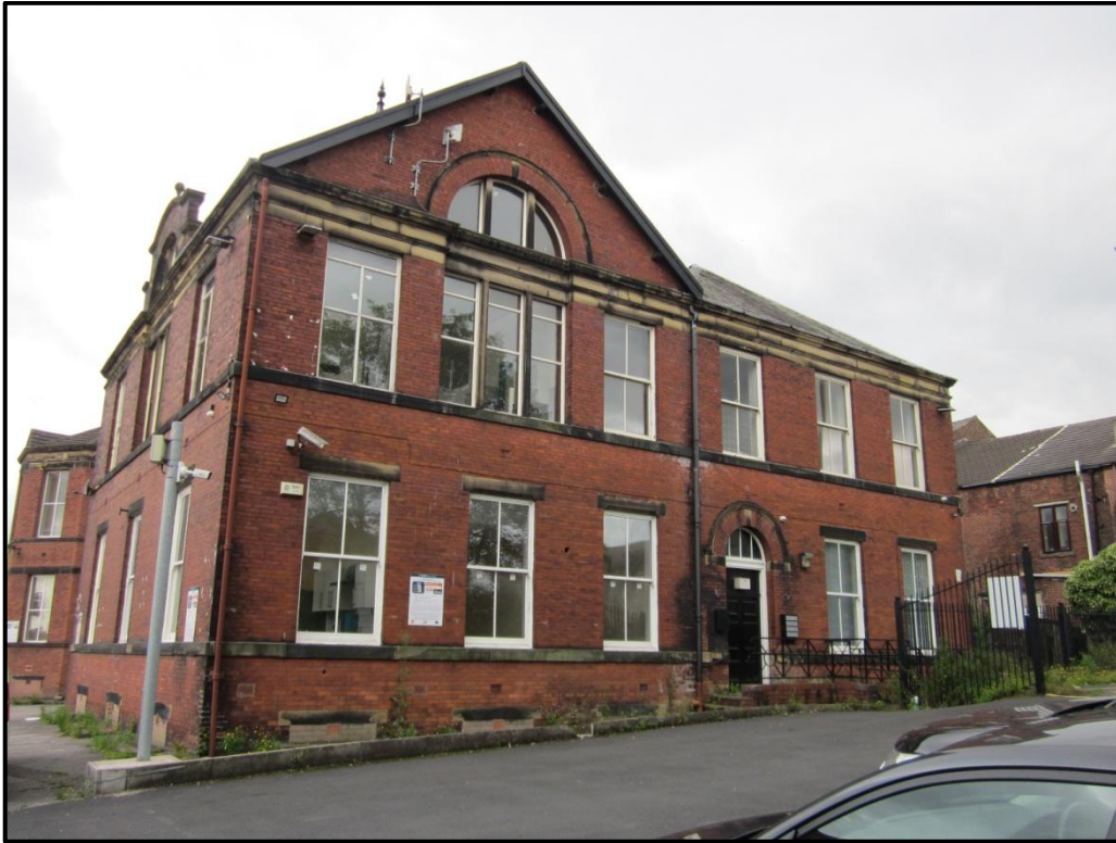
Photograph 1. Former council offices, 150 Yorkshire Street
