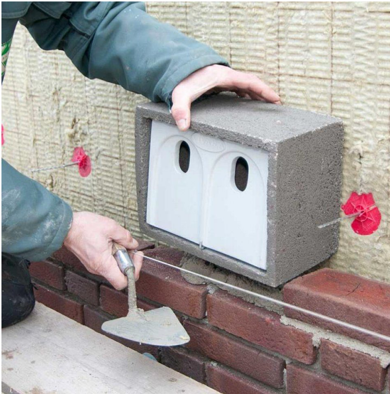
Figure 4 – Example Build-in Sparrow Terrace 5
