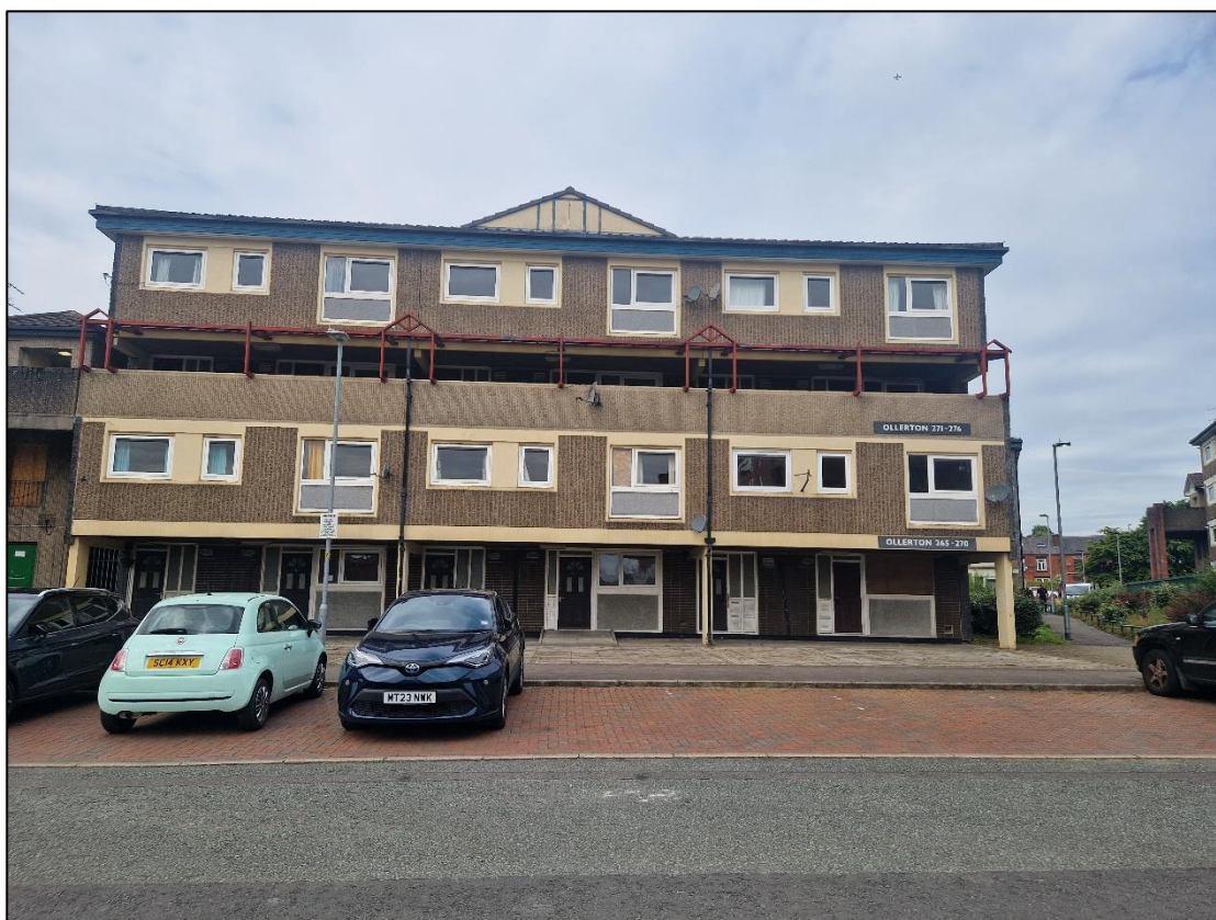
Plate 1 – Character of buildings on site
