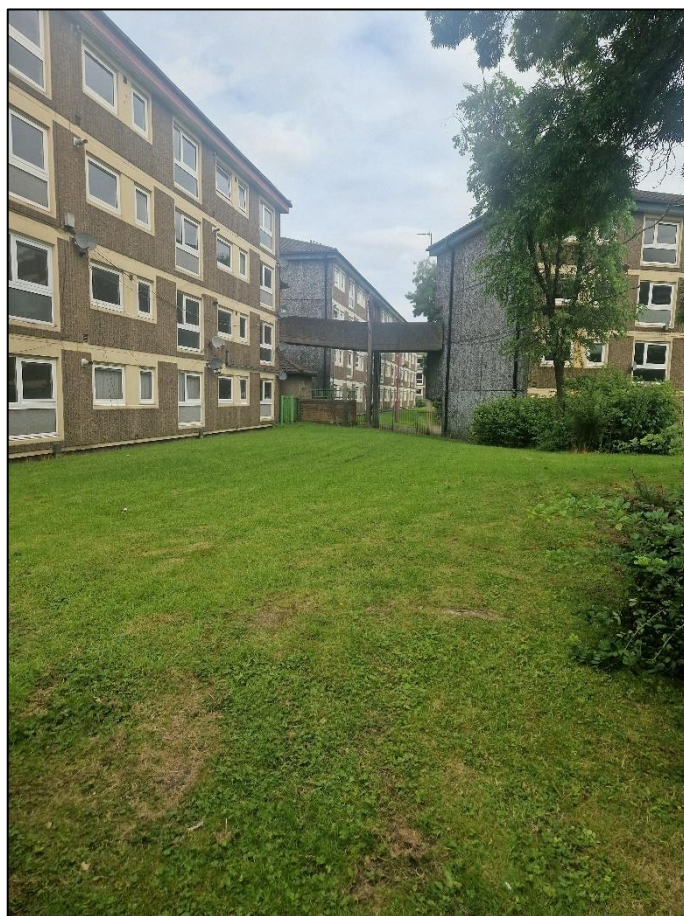
Plate 3 – Character of site
