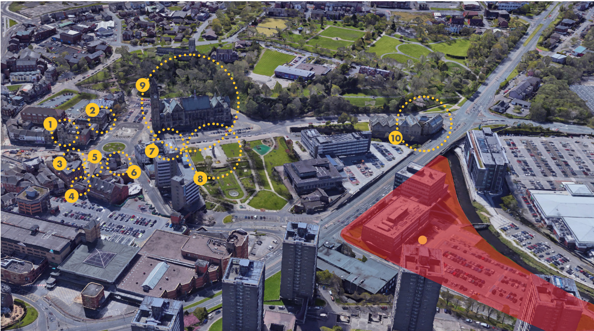
Aerial view of area of Rochdale around the Town Hall. Image courtesy of Google Earth.
