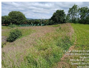
Embankment in the west of the site
