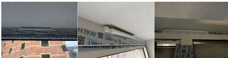
Figure 3 – Windows Closed and Vents Opened
