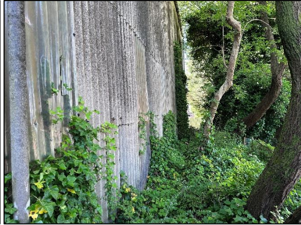
Figure 19: The tree line to the rear of the building.
