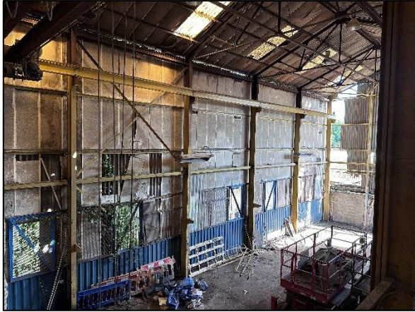
Figure 18: The interior of Area 2, viewed from Area 1.
