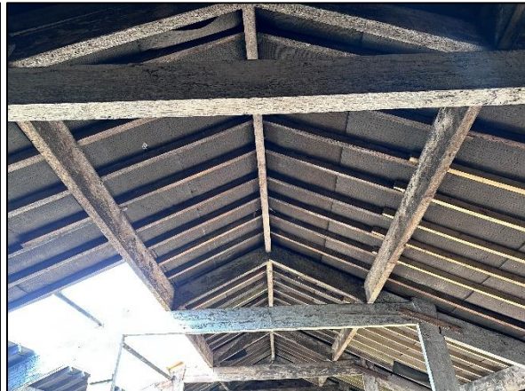
Figure 15: The bituminous lining felt present in Area 1.
