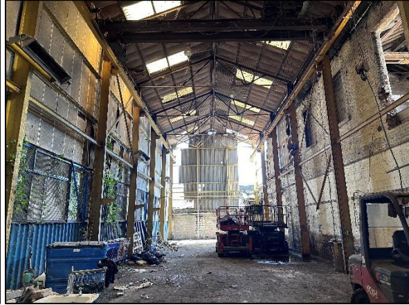
Figure 6: The interior of Area 2.
