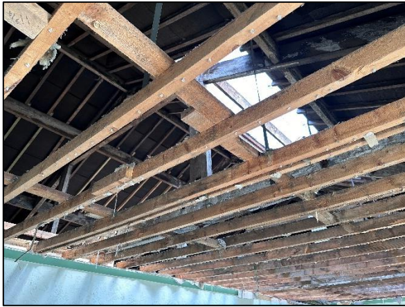
Figure 8: Removed ceilings within Area 1.
