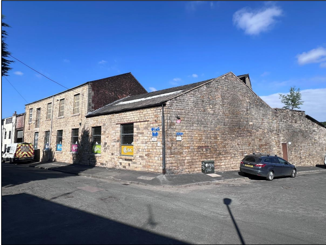
Figure 2: Area 1 of the building, viewed from the northeast.
