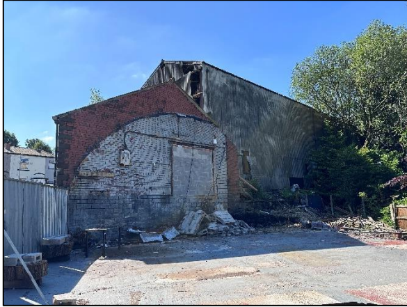
Figure 5: Area 2, the large metal framed structure.
