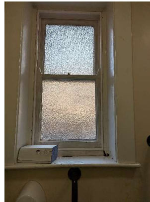
First repaired windows re-installed
