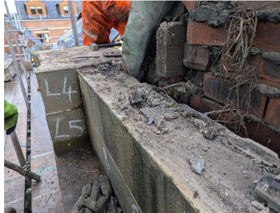
All stonework referenced and identified on a reference drawing before dismantling
