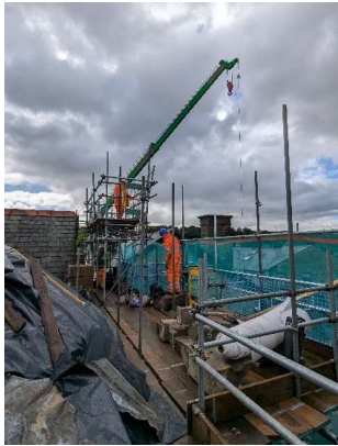
Crane used to dismantle upper stonework of entrance from the entrance gable and oriel window
