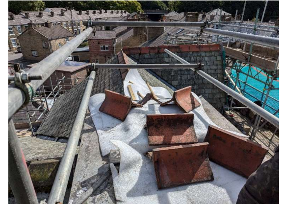
Roof cowel removed for repair
