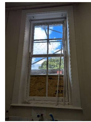
Repaired kitchen window re-installed
