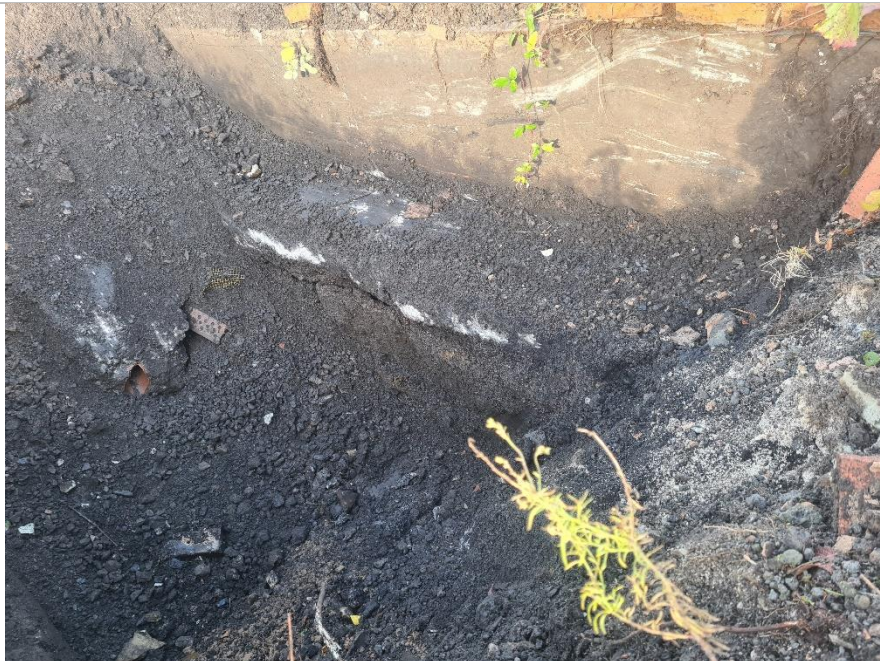
EXPOSED FOUNDATION – TP307
