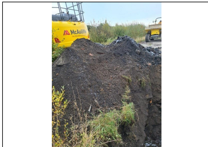
TP211 East spoil
