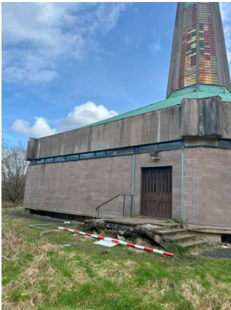
Rear steps to be retained and repaired
