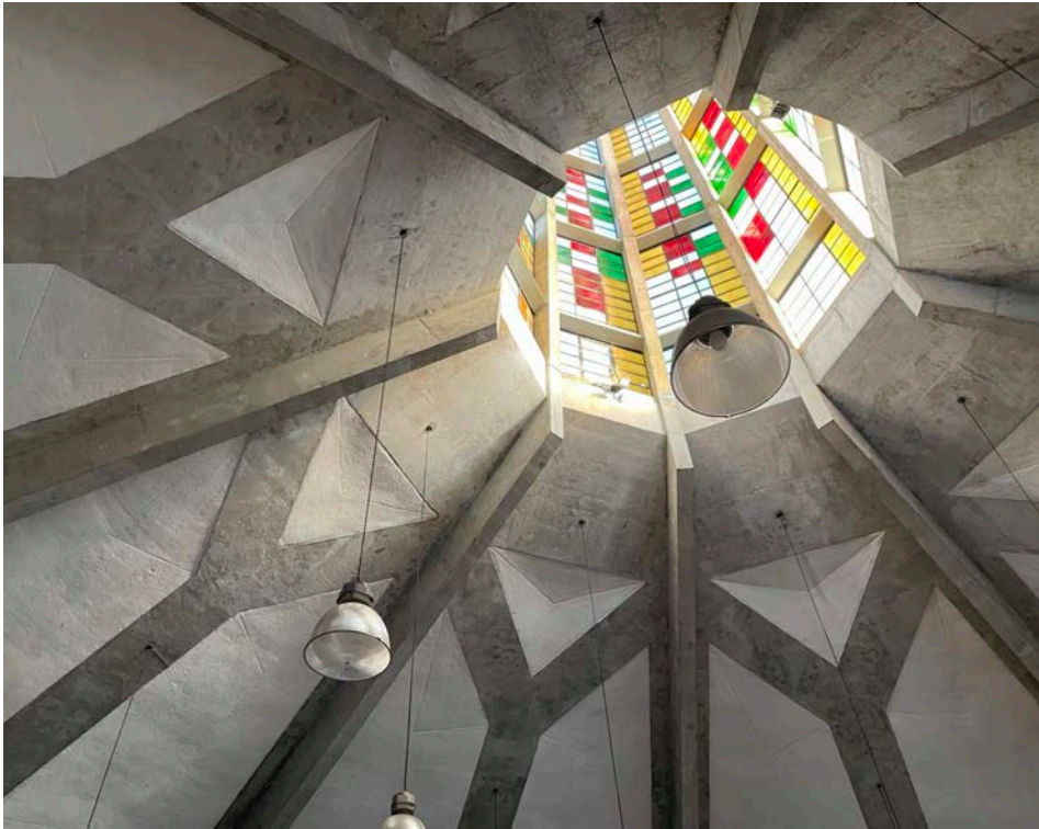
1 View looking up towards stain glass window.
