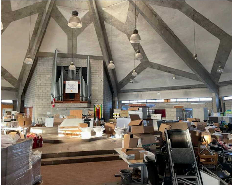
2 View into the main hall, currently being used for storage.
