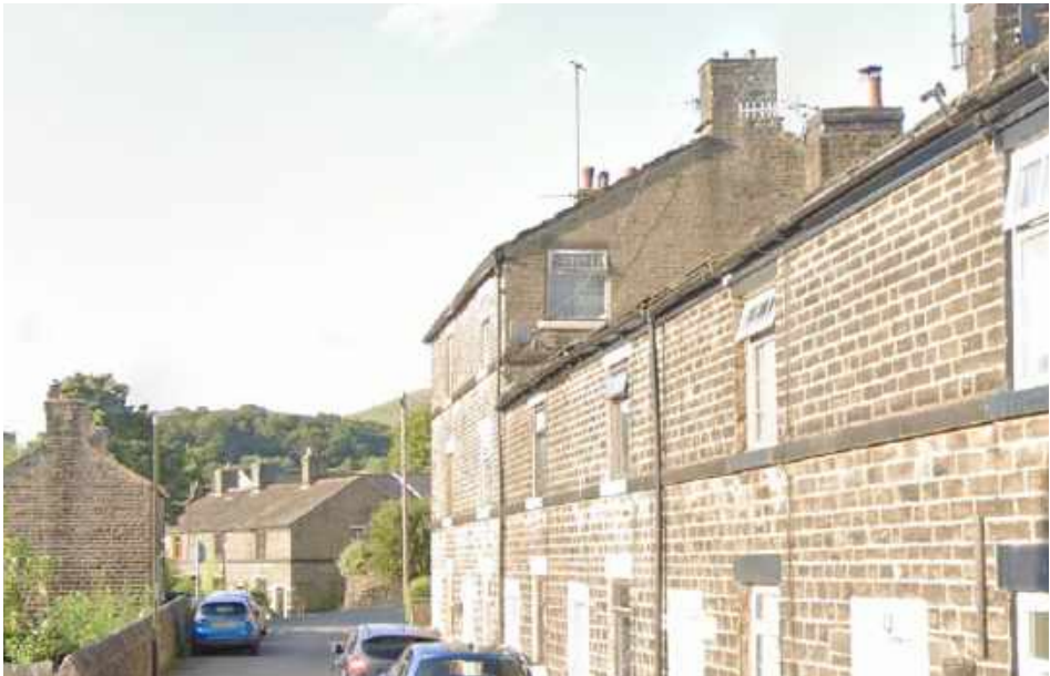
Prominent chimney gables and stepping up to corner (old glossop)
