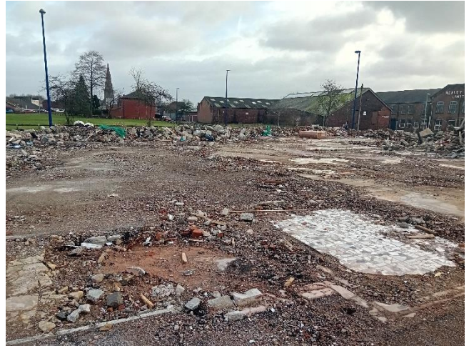
Photo 2: Developed land; sealed surface on the site of the former building.
