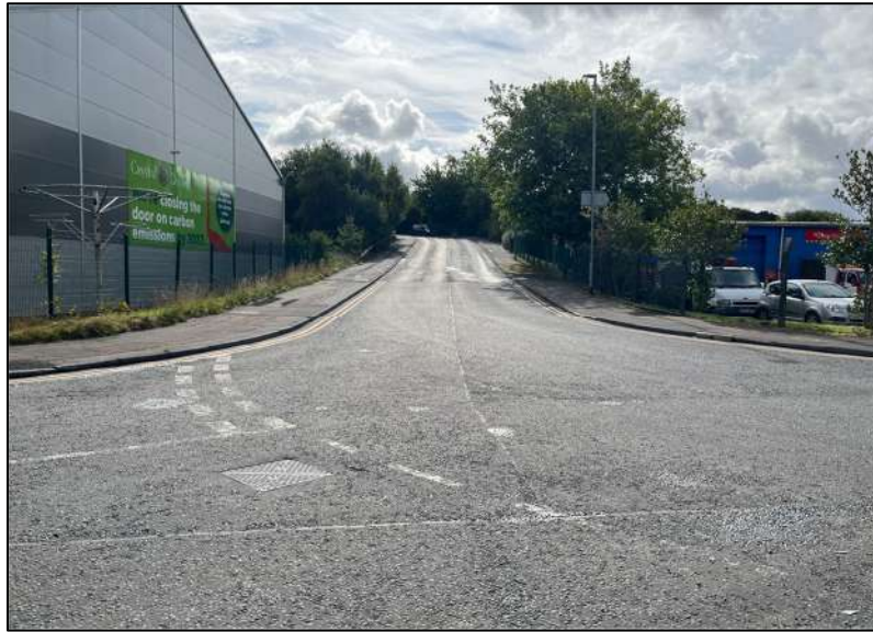
Plate TS7 - Gorrells Way / Hanson Place Junction Looking Towards Canal Bridge on Gorrells Way
