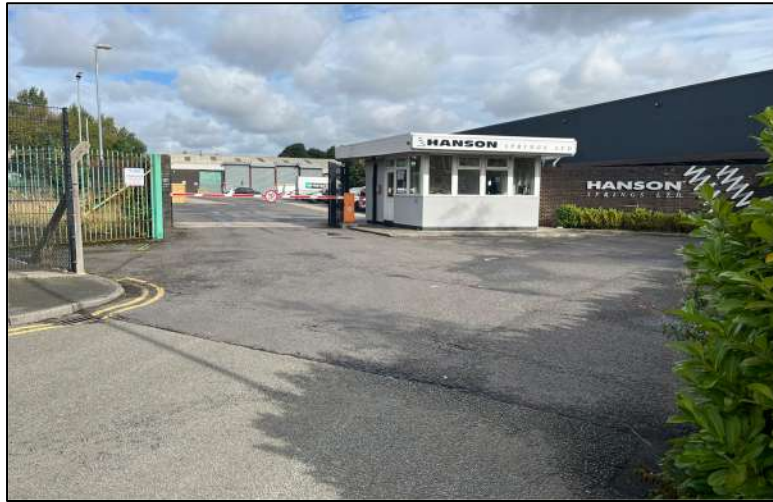
Plate TS4 - Hanson Springs Site Entrance and Security Lodge
