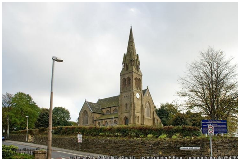
FIG 02 A Grade II Listed Building in Castleton, Rochdale,
