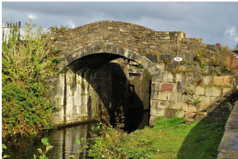
FIG 01 Rochdale Canal Lock Number 52 and Towpath
