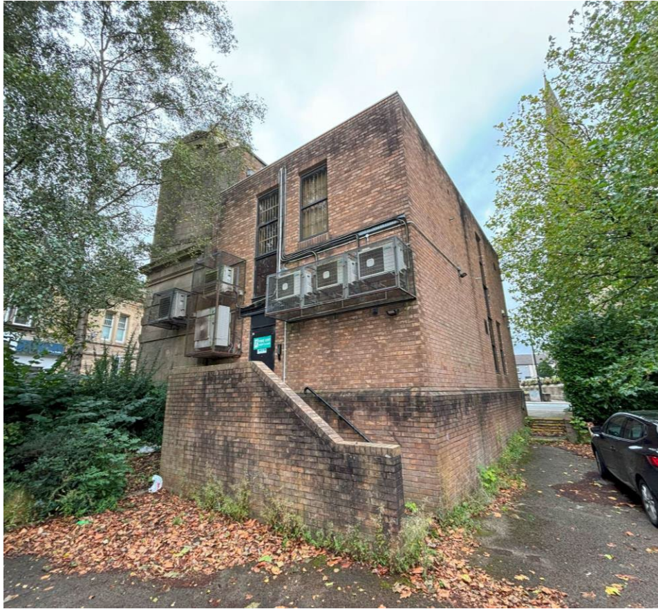
Figure 3 Grade II Listed 2 Church Street Extension showing three condensers on the right to be removed and replaced with one condenser
