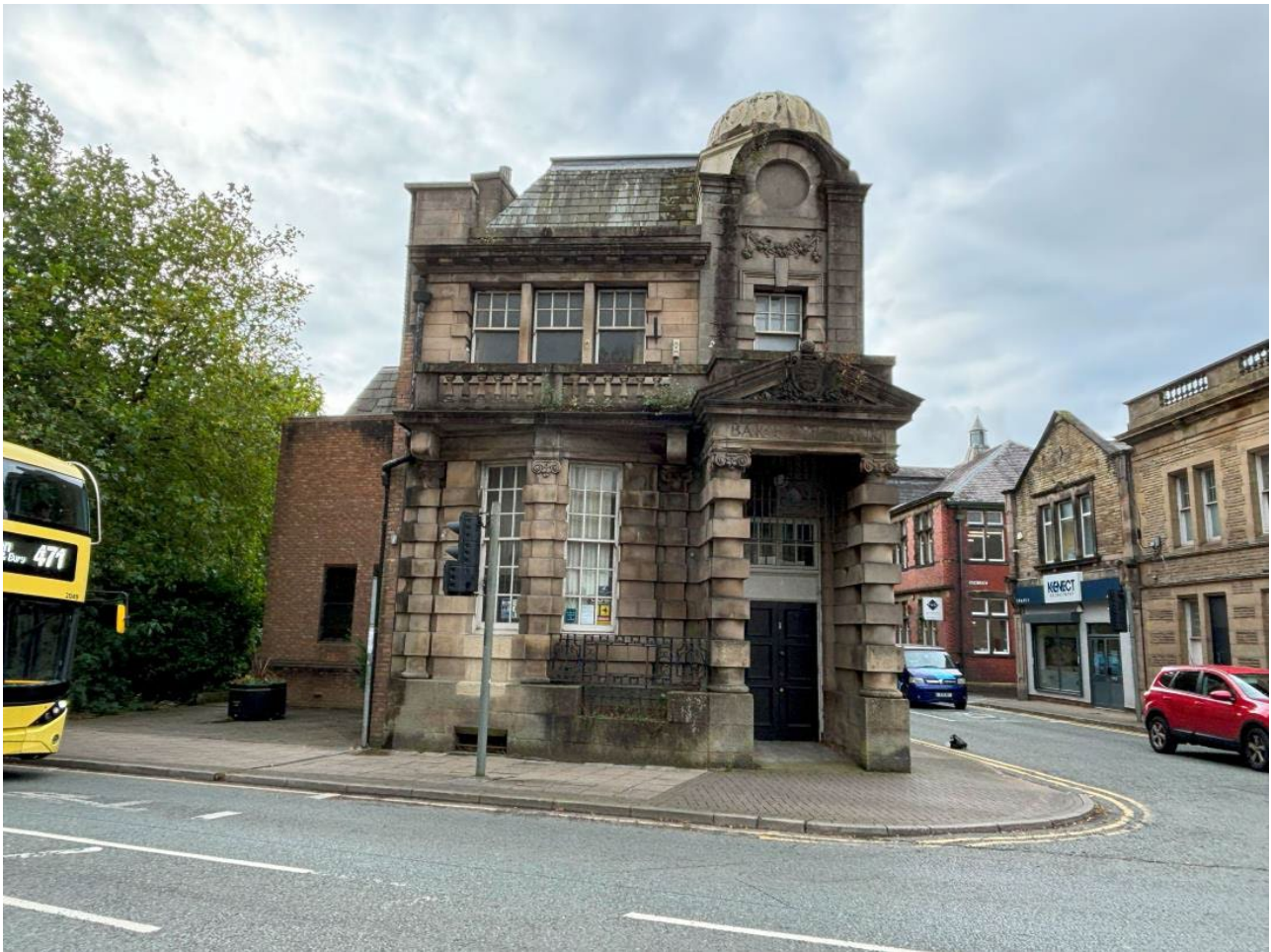
Figure 1 Grade II Listed 2 Church Street Front Elevation
