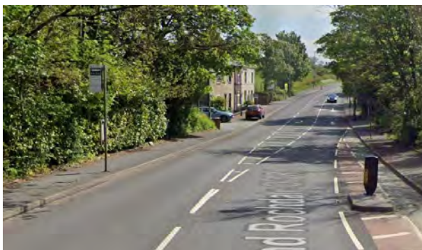
Plate 2: Eastbound Bus Stop
