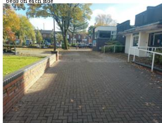
Photograph 8: Viewing East to West ul b6-1 adjacent to Heywood Civic Centre
