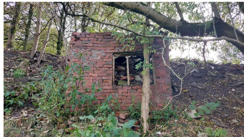
Photograph 8: Derelict building on the site's northern boundary. Building was of negligible suitability to support bats.
