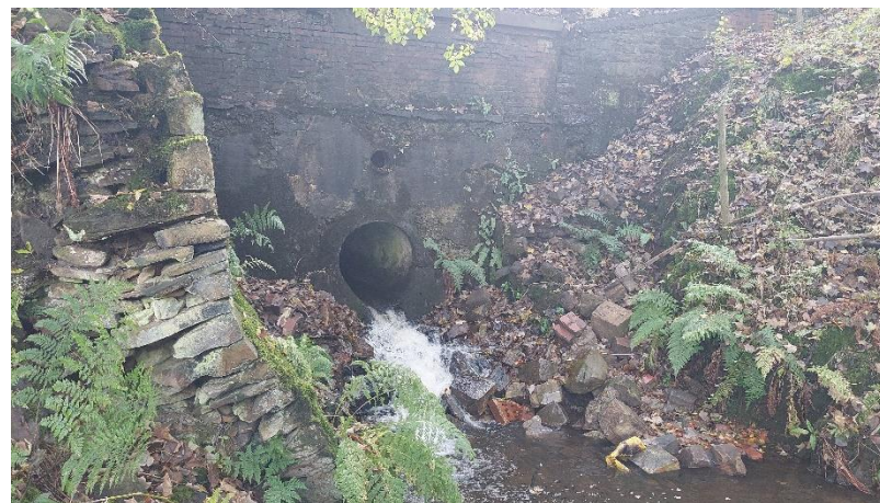
Photograph 10: Cylindrical culvert on the site's northern boundary.
