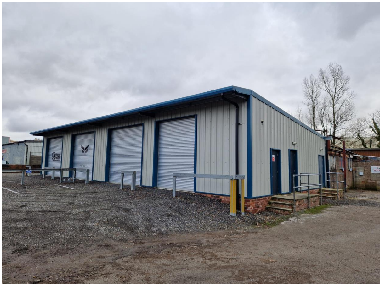
[Above – Photograph of existing units 4 & 5, which the proposals seek to replicate]
