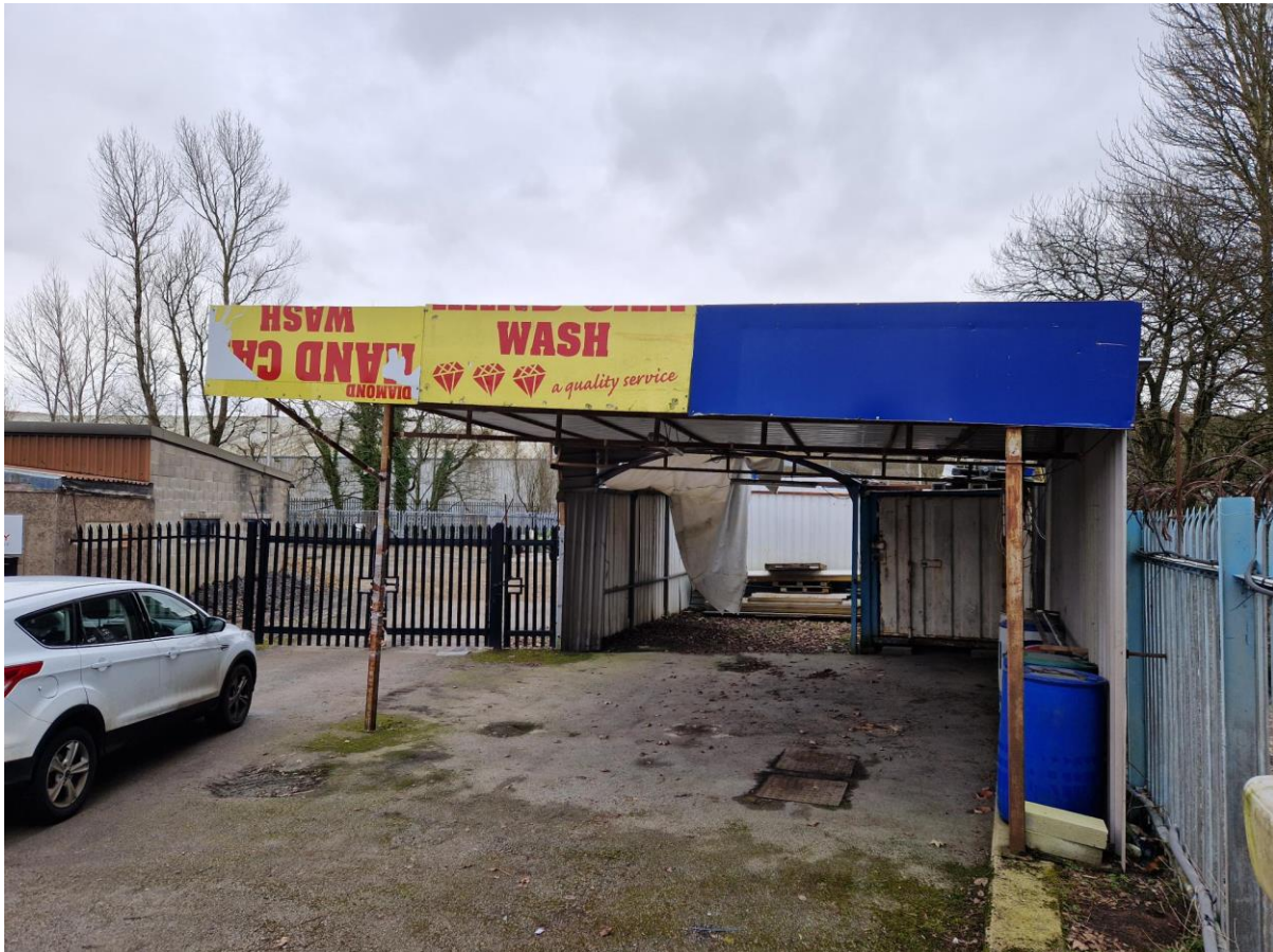
[Above – Photograph of the covered former car wash proposed to be demolished]
