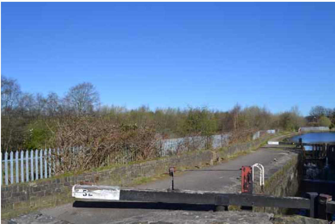
Plate 30: Sightline to the north-west from the Rochdale Canal Lock No. 52 and Towpath Bridge (Listed Building Grade II, NHLE ref. 1038295)
