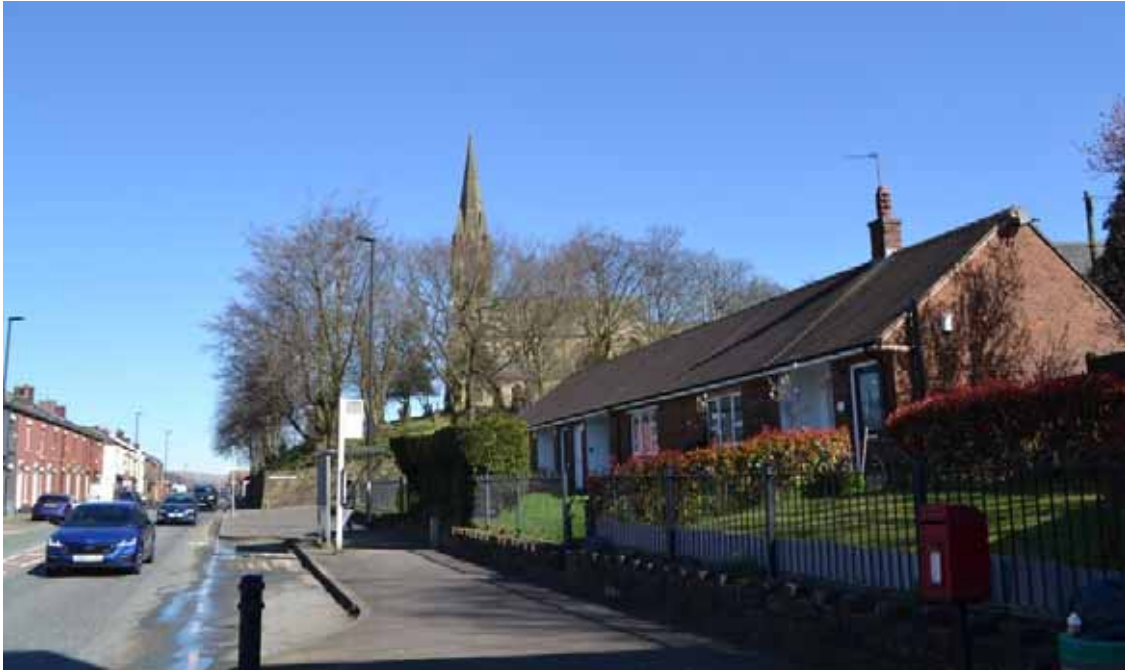
Plate 43: Sightline to the north along A664 Manchester Road within the Castleton South Conservation Area. Tower and spire of St. Martin's Church (Grade II, NHLE ref. 1203230)) is prominent. The proposed development would have no visual influence on this sightline. This is a 'Key View' within the Conservation Area. The proposed development would have no visual influence on this sightline
