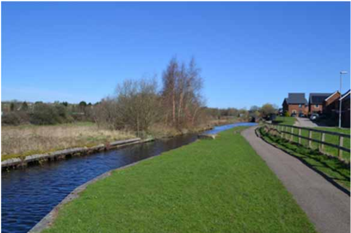
Plate 36: Sightline to the north from Rochdale Canal Lock No. 53 (Grade II, NHLE ref. 1346237)
