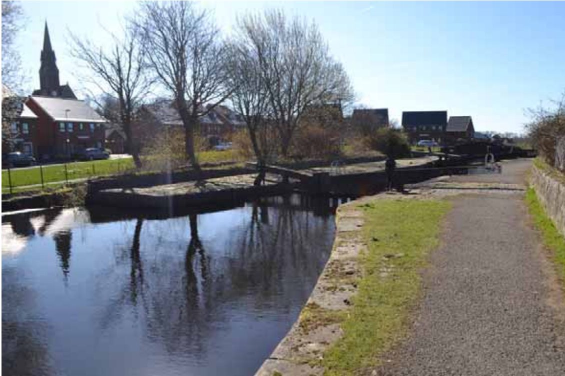
Plate 29: Sightline to the south towards the Rochdale Canal Lock No. 52 and Towpath Bridge (Listed Building Grade II, NHLE ref. 1038295)
