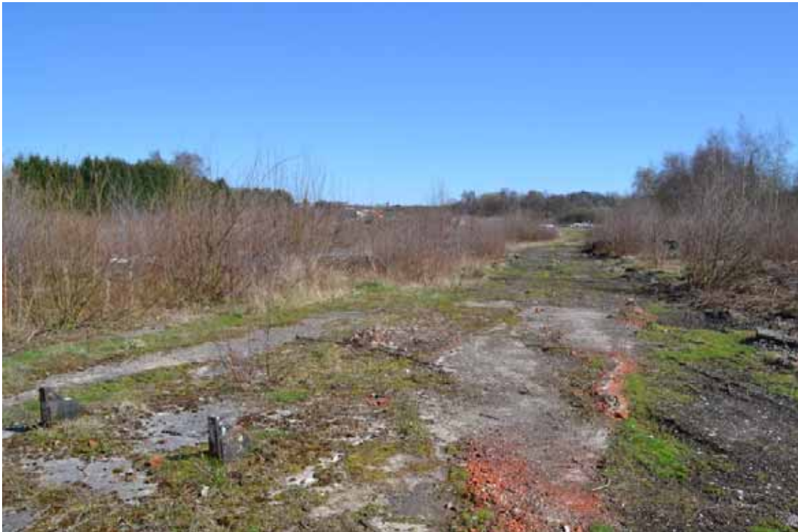
Plate 13: Sightline to the east across the Site showing degraded hardstanding.
