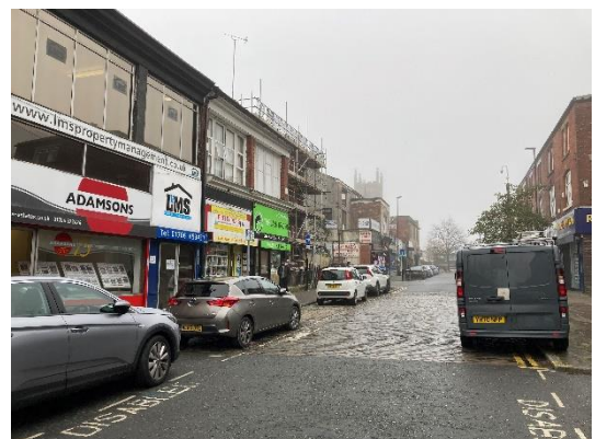
Fig 6: Signage in the conservation area on Yorkshire St.
