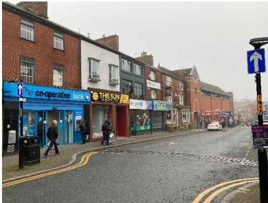
Fig 7: Signage in the conservation area on Yorkshire St.
