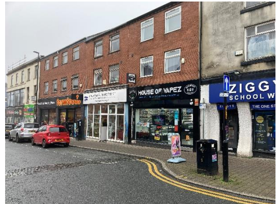
Fig 8: Signage in the conservation area on Yorkshire St.
