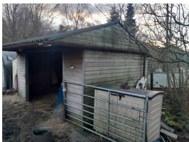
Photo 4: Building one, viewed from the northwest.
