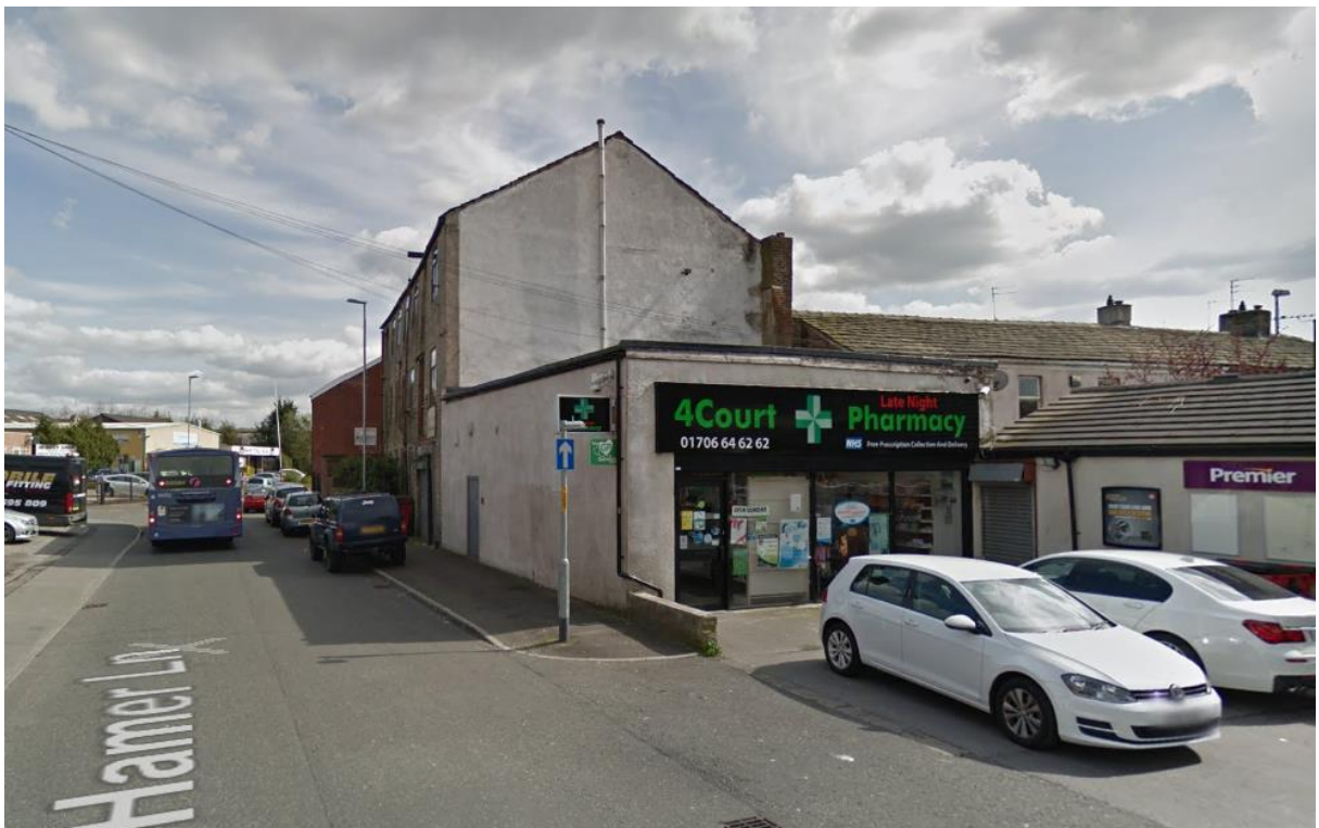
Above: Existing flat roofed rendered Pharmacy building.
