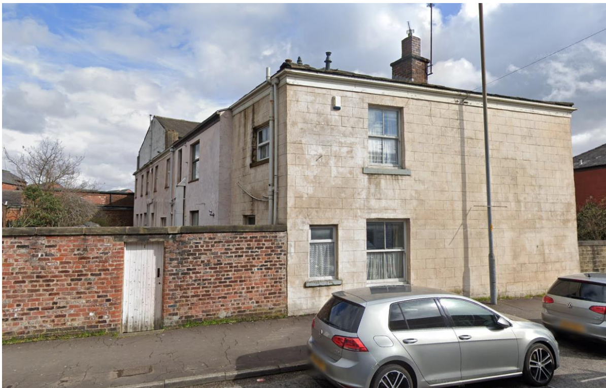
Above: Rear and gable elevations of Heybrook House flats today.
