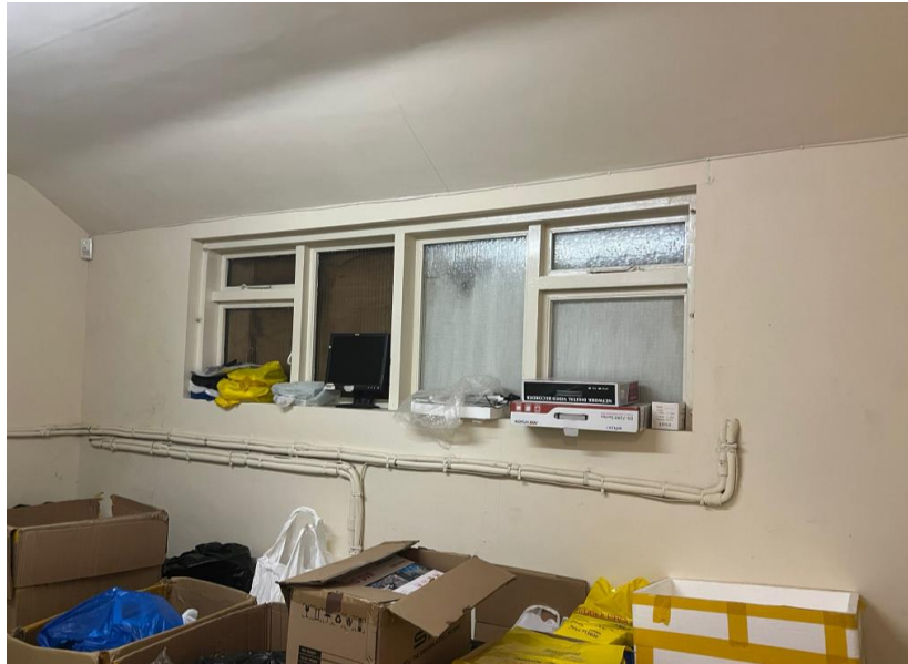
Above: Rear upper floor window boarded up externally, this will be opened up and original window retained.
