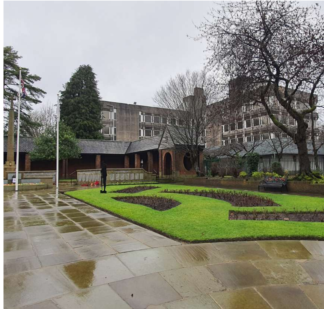
View of the existing Parkfield House from the Garden of Remembrance
