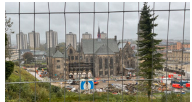
3.19 The Site fully visible over the 'Saxon' Wall
