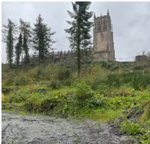
3.23 View towards the 'Saxon' Wall (obscured by vegetation and not accessible due to tree works)
