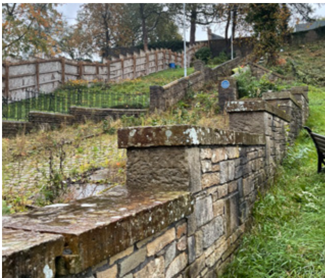
3.44 East boundary wall to Packer Spout Gardens, meeting the older wall of Church Steps
