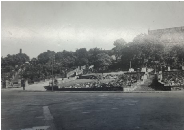
2.38 Packer Spout Gardens, the entrance to Church Steps adjacent formed the surviving remnant of Packer Street, c.1935 (Rochdale Local Studies)
