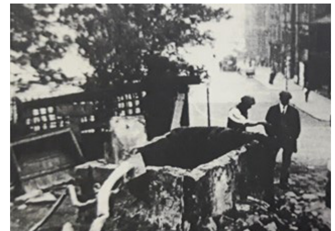
2.47 Water tank system, Packer Street, c.1926-27 (Rochdale Local Studies)
