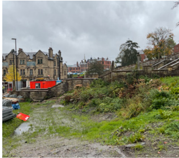
3.51 West garden area, terracing part surviving closest to the built feature, with remnant planting
