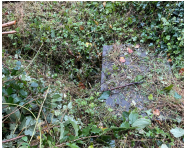
3.40 Modern basic drainage channel, reusing found stone
