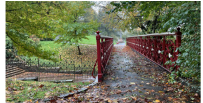
3.9 Broadfield Slopes, Victoria Bridge
