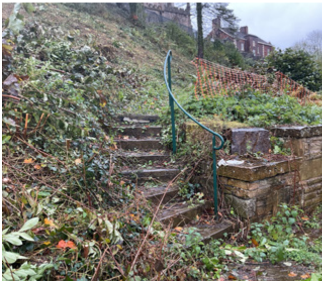
3.61 Retaining wall with modern steps running up to The Slopes
