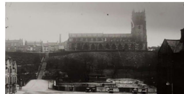
2.35 The Slopes during demolition of the corn mill, 1931 (RDA)
