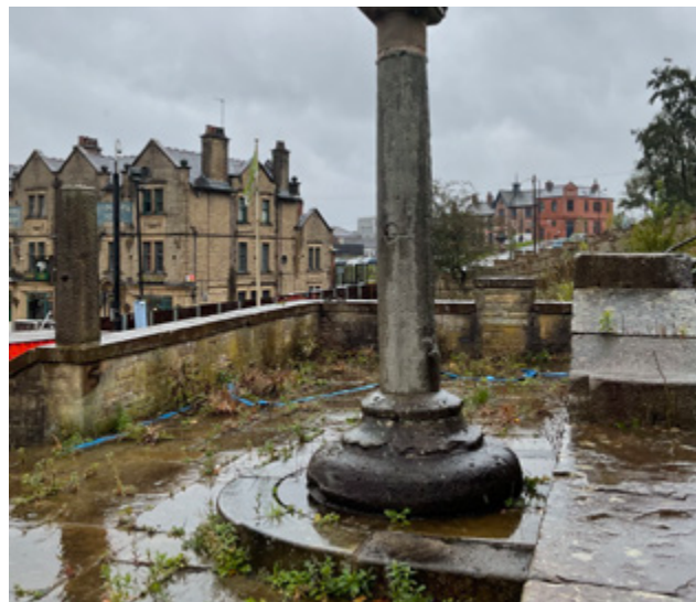
3.58 Market cross shaft, with a later finial and a base of unknown date
