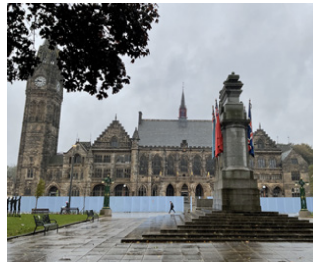
3.1 Front of Rochdale Town Hall, viewed from the Cenotaph and Memorial Gardens to the north
