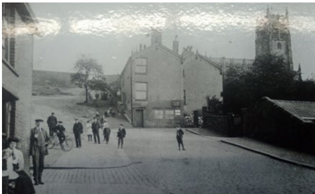
2.26 Packer Street (leading to Church Steps), with buildings along The Slopes (R) (Rochdale Local Studies)
