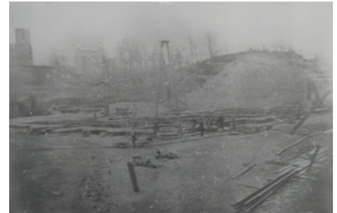
2.25 Town Hall under construction in the north of The Slopes, 1866 (Rochdale Local Studies)
