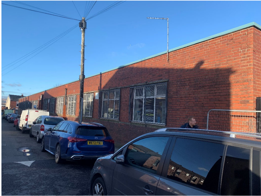
View of Smalley Street elevation
