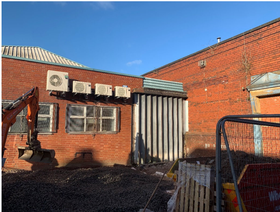
Side view showing existing shutter to be replaced
