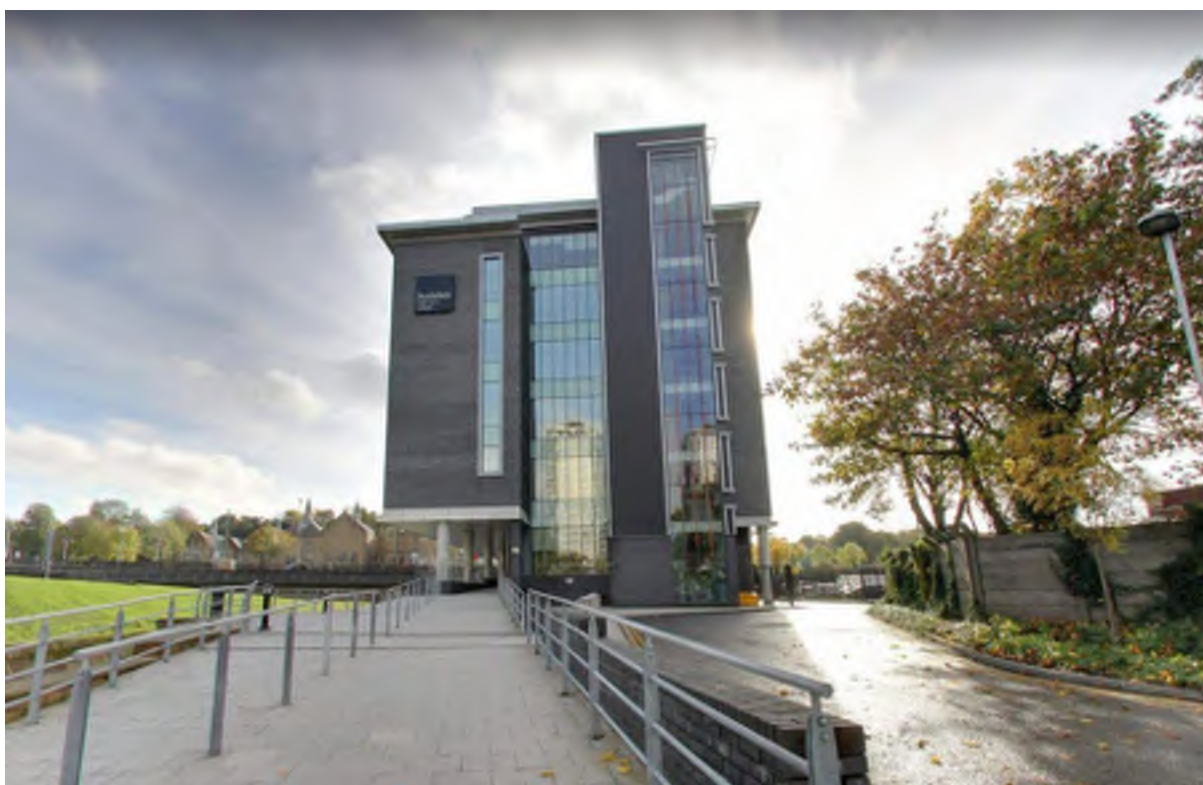
Plate 6: View of the southeastern end of the Site with the existing Rochdale 6 th Form College building beyond.
