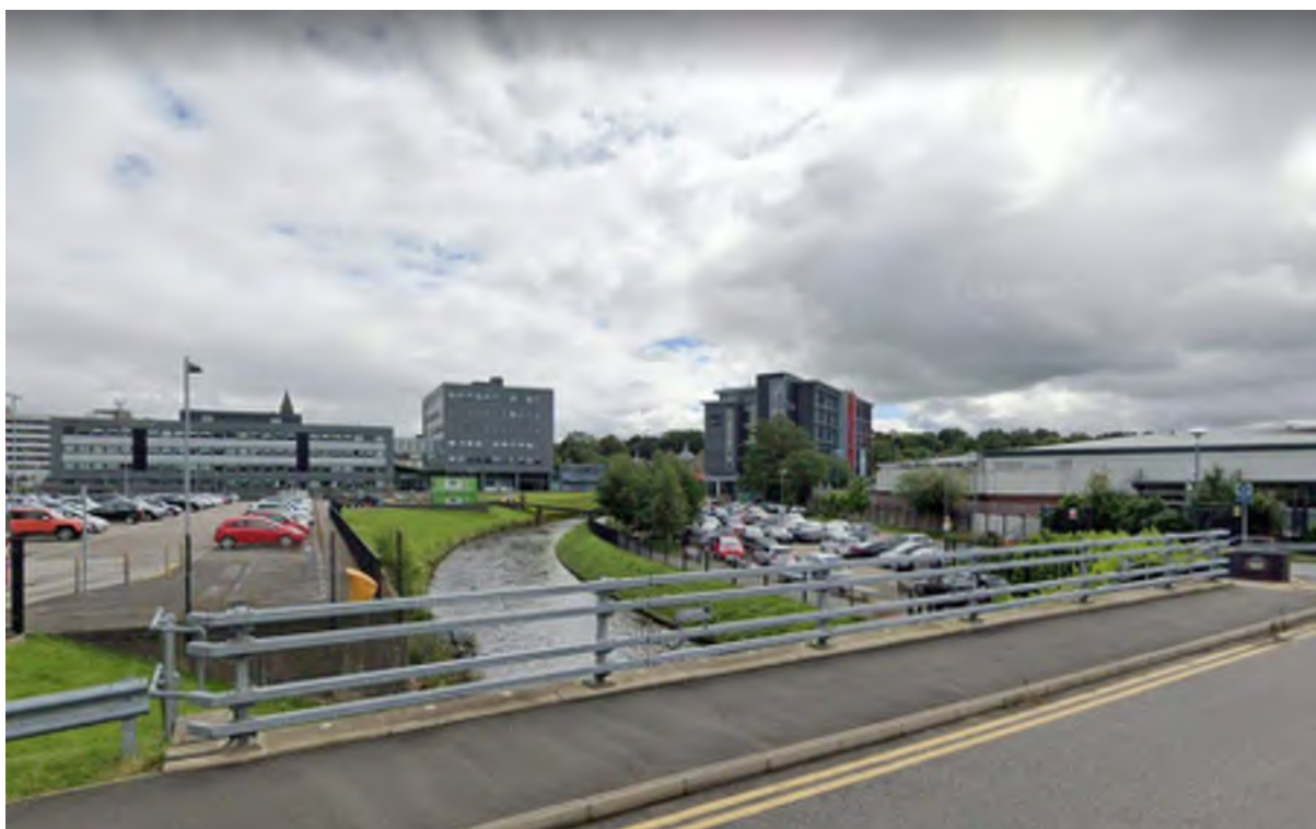
Plate 3: View of the River Roch channel from the bridge at the west of the Site
