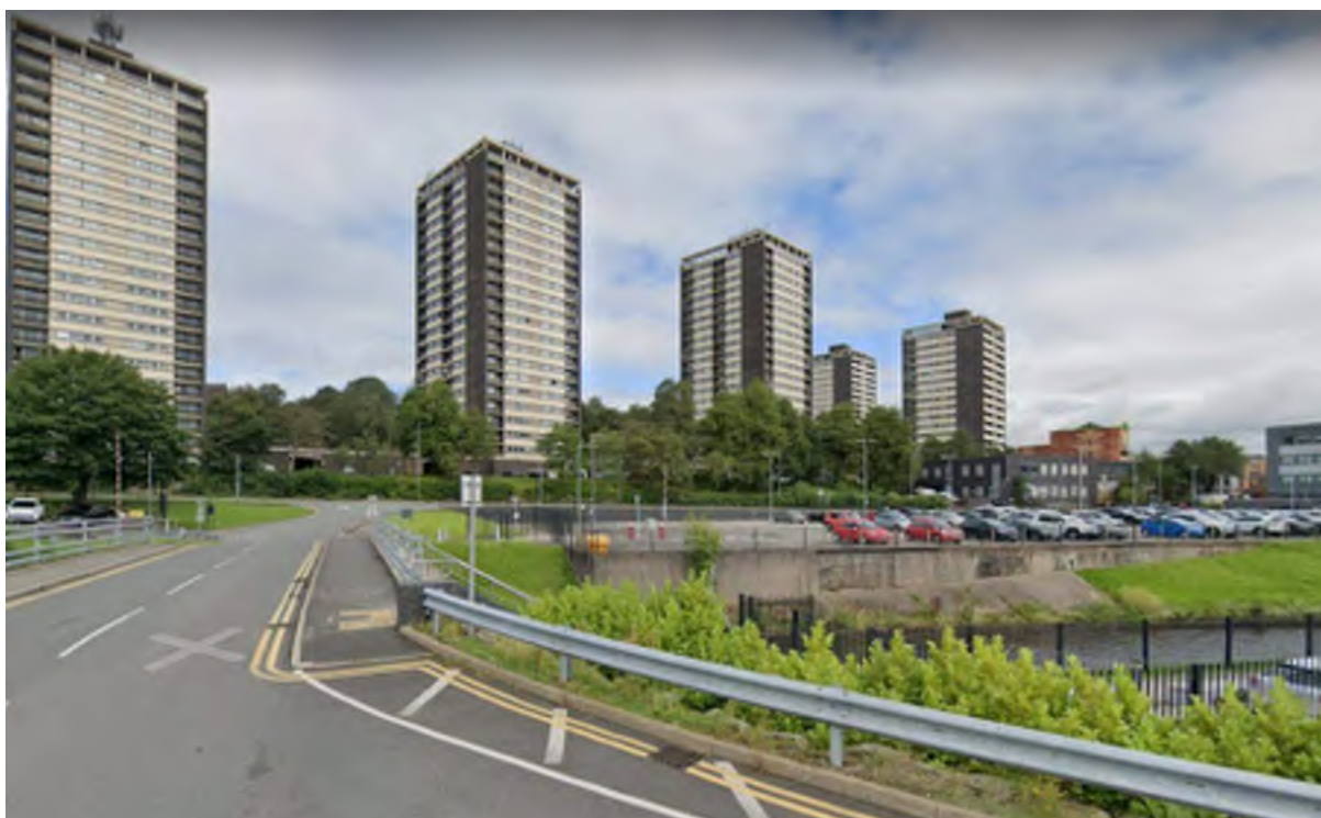
Plate 1: View of the bridge over the River Roch at the western end of the Site
