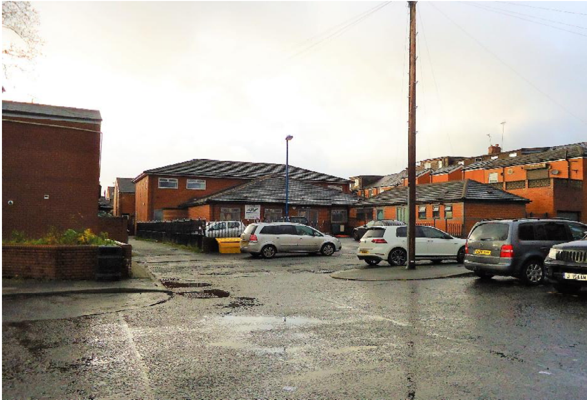
The image above is the rear and side elevation of the application property located on Aboukir Street with a small car park in front of the building.
