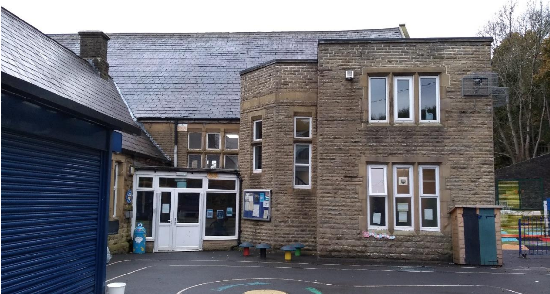
Figure 3: Existing main entrance.
