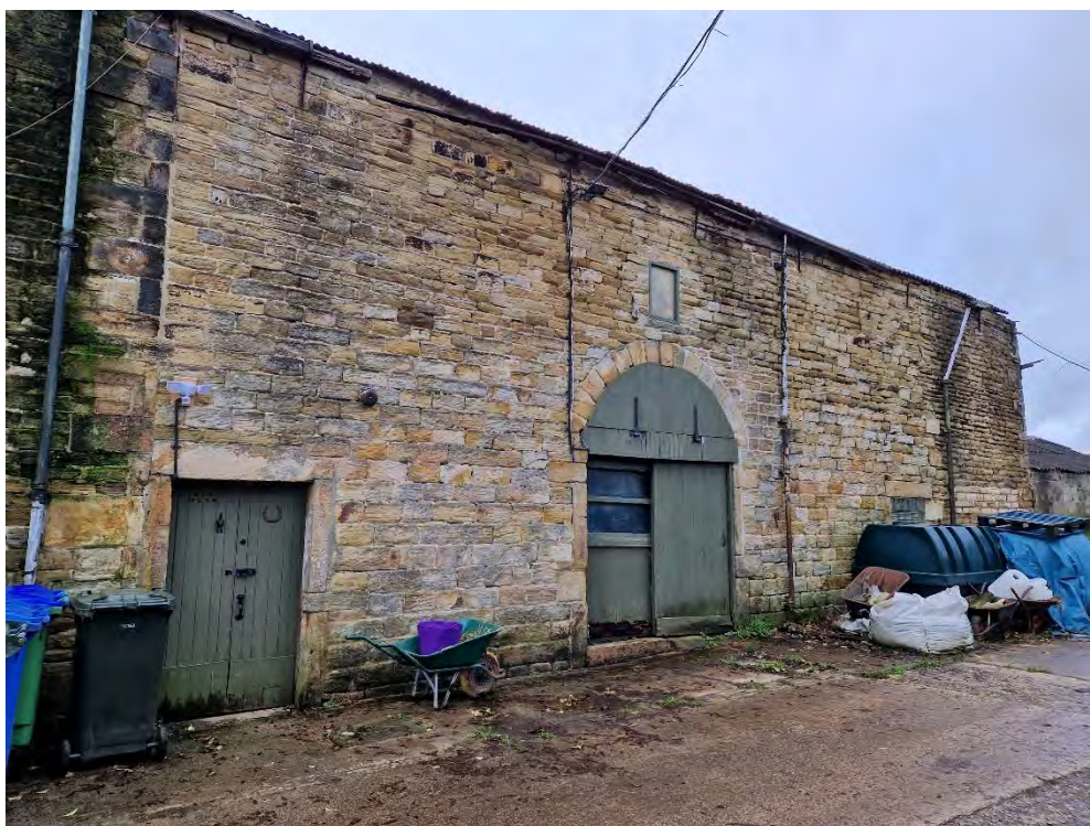
Plate 2: Lower Cleggswood Farm barn - building C (north-eastern elevation), looking north-west
