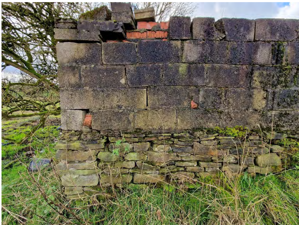
Plate 13: Structural remains at Heald Spring, looking south
