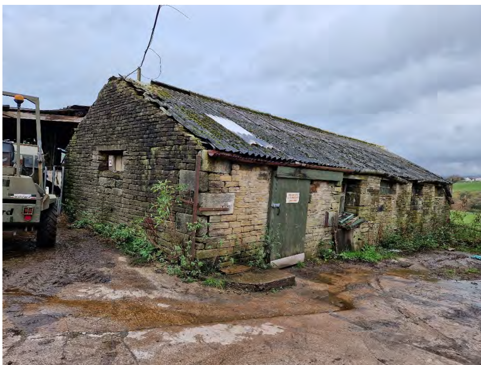
Plate 4: Lower Cleggswood Farm outbuilding - building G (south-western and south-eastern elevations), looking north
