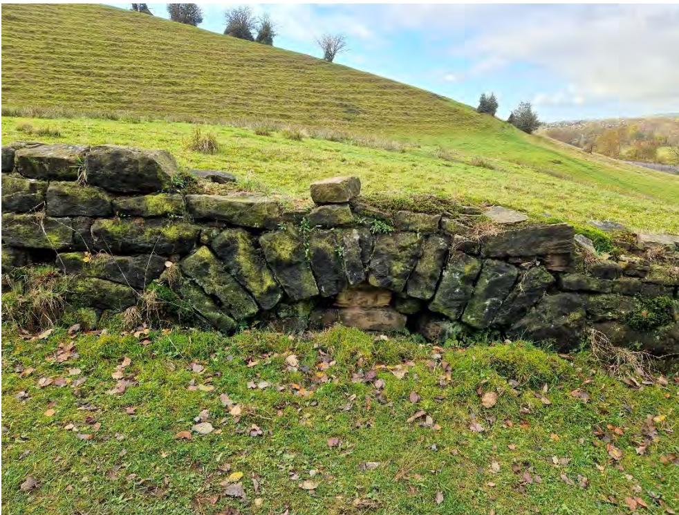
Plate 6: Drystone wall along western edge of Heald Lane including remains of an arched opening, looking west
