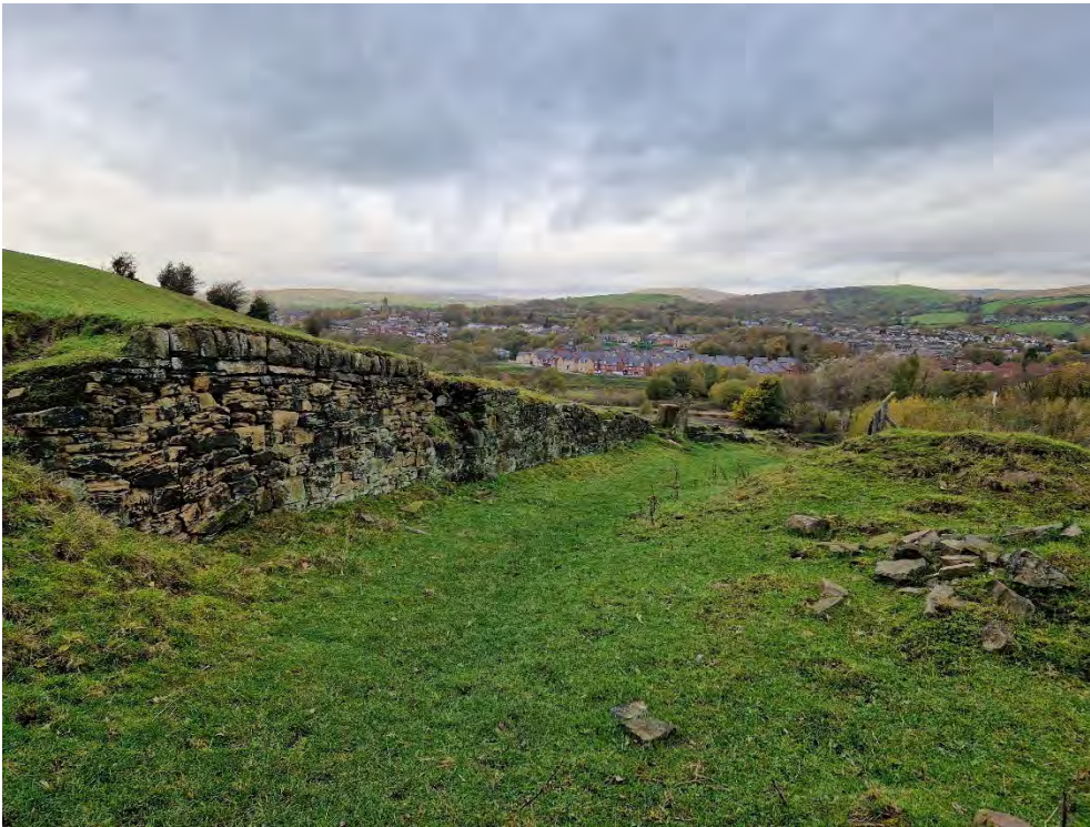
Plate 5: Drystone wall along western edge of Heald Lane opposite former cottages at Brown Bank Top, looking north-west
