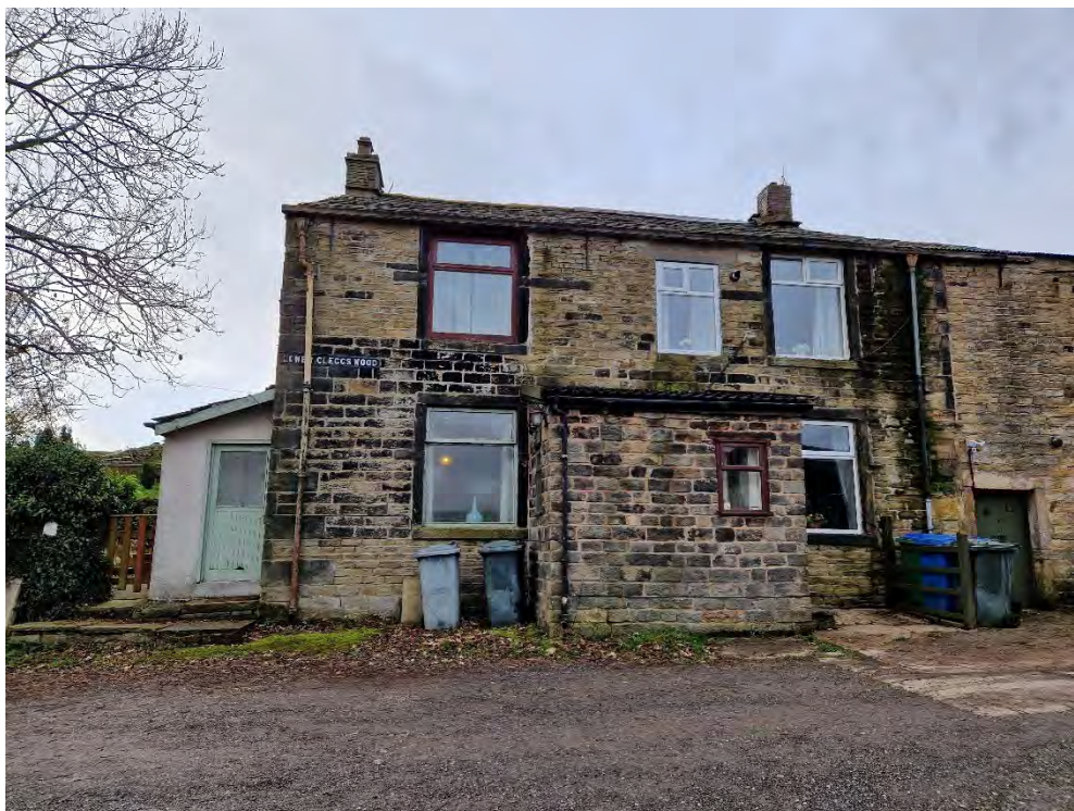
Plate 1: Lower Cleggswood Farm cottages - building A & B (north-eastern elevation), looking south-west
