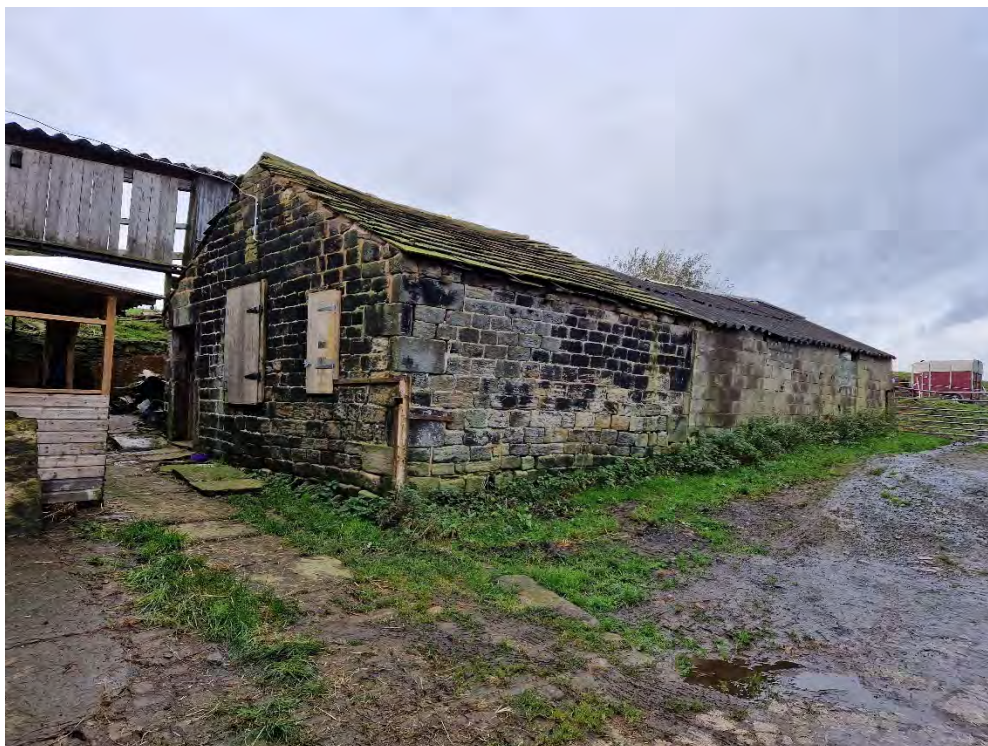
Plate 3: Lower Cleggswood Farm outbuilding - building D (north-eastern and south-eastern elevations), looking west
