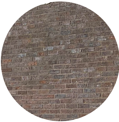
EXISTING BRICK TEXTURE
