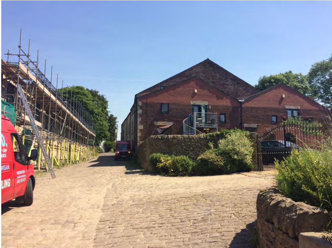
Plate 17: Clegg Hall Mill complex. The earliest building is on the right and the rebuilt Canalside Mill range is on the left.
