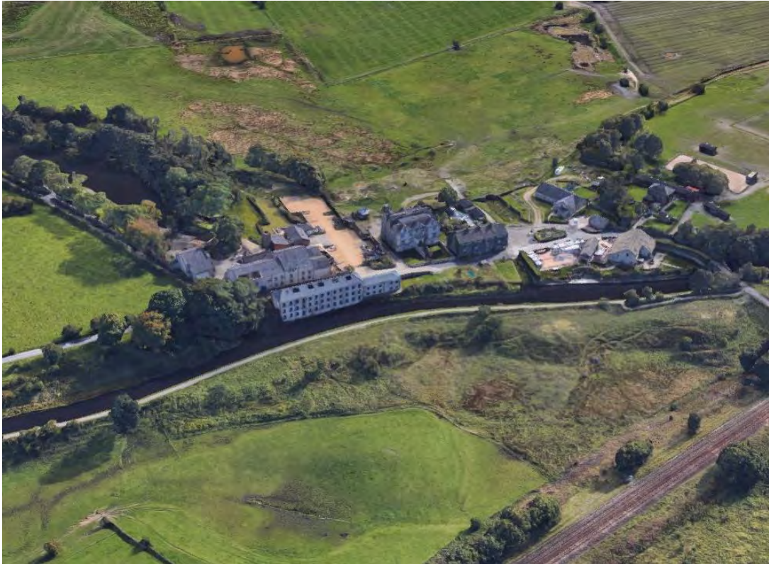
Plate 21: South facing aerial view of Clegg Village Conservation Area, showing the rebuilt and restored Clegg Hall Mill complex.
