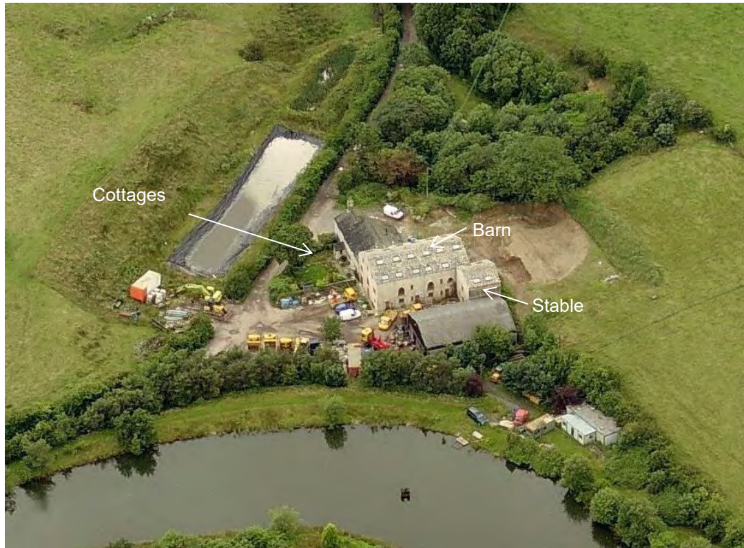
Plate 25: West facing aerial view of Lower Eafield Cottages, Barn and Stables.
