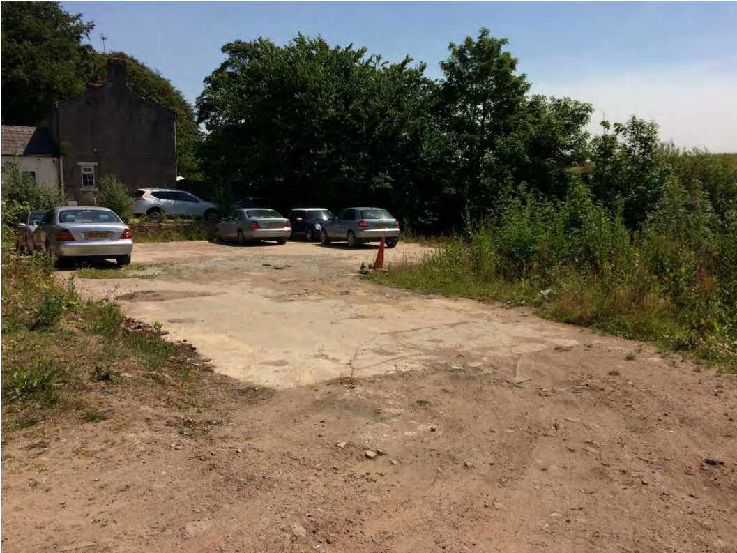
Plate 29: Hardstanding remains of the hand-loom weaving shed.
