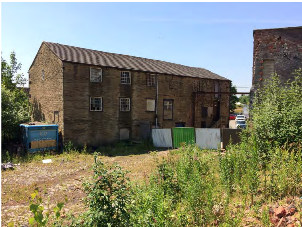
Plate 26: South facing view of the late 18th century mill building, Grade II listed Dob Wheel Mill.
