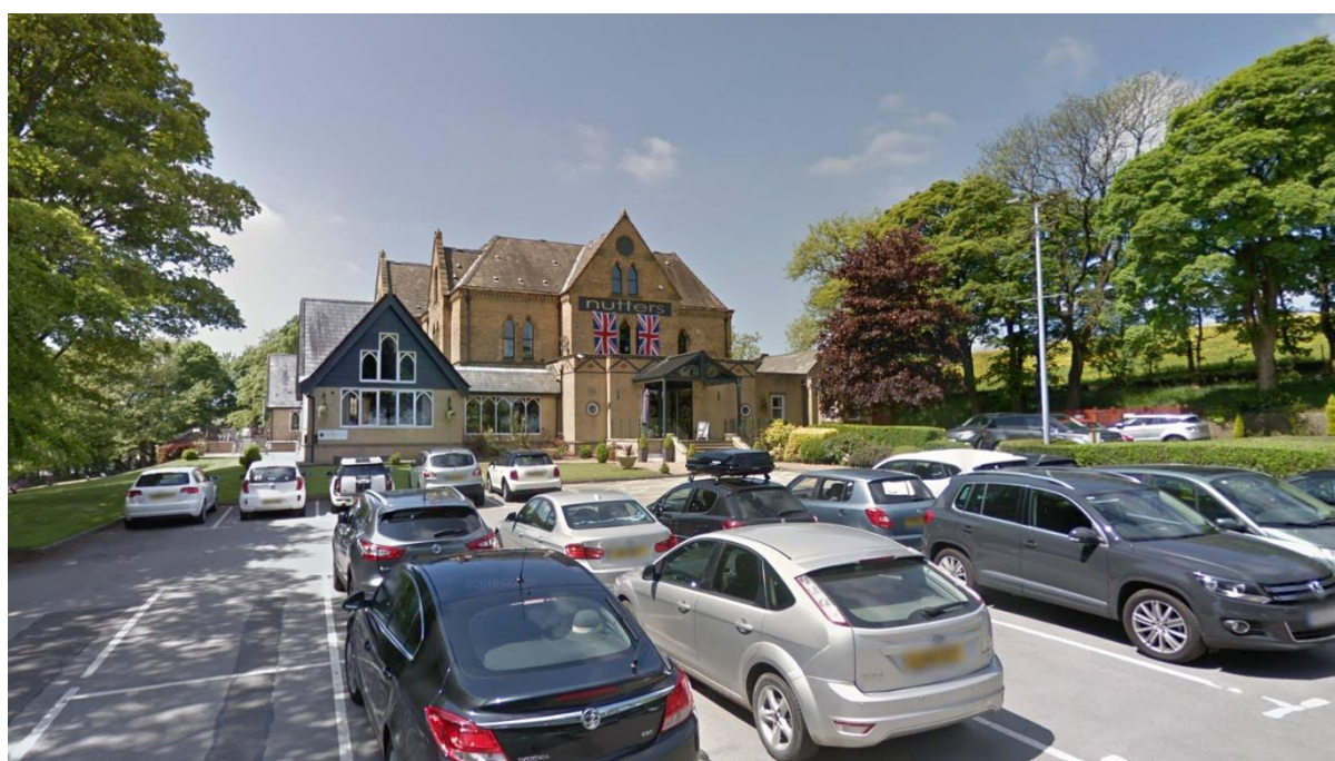
Figure 6. Image of the east facing elevation. The modern extensions clearly designed with an intention of replicating the architecture of the building.
