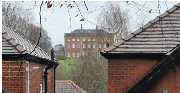
5. View of Alkrington Hall from the elevated grounds of Parkfield House
