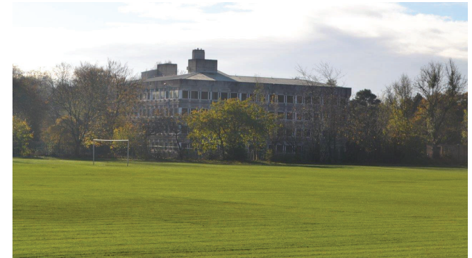
4. View from Limefield Leisure Park
