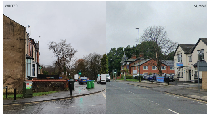
1. Gateway entry into the CA from the east - Middleton Town centre
