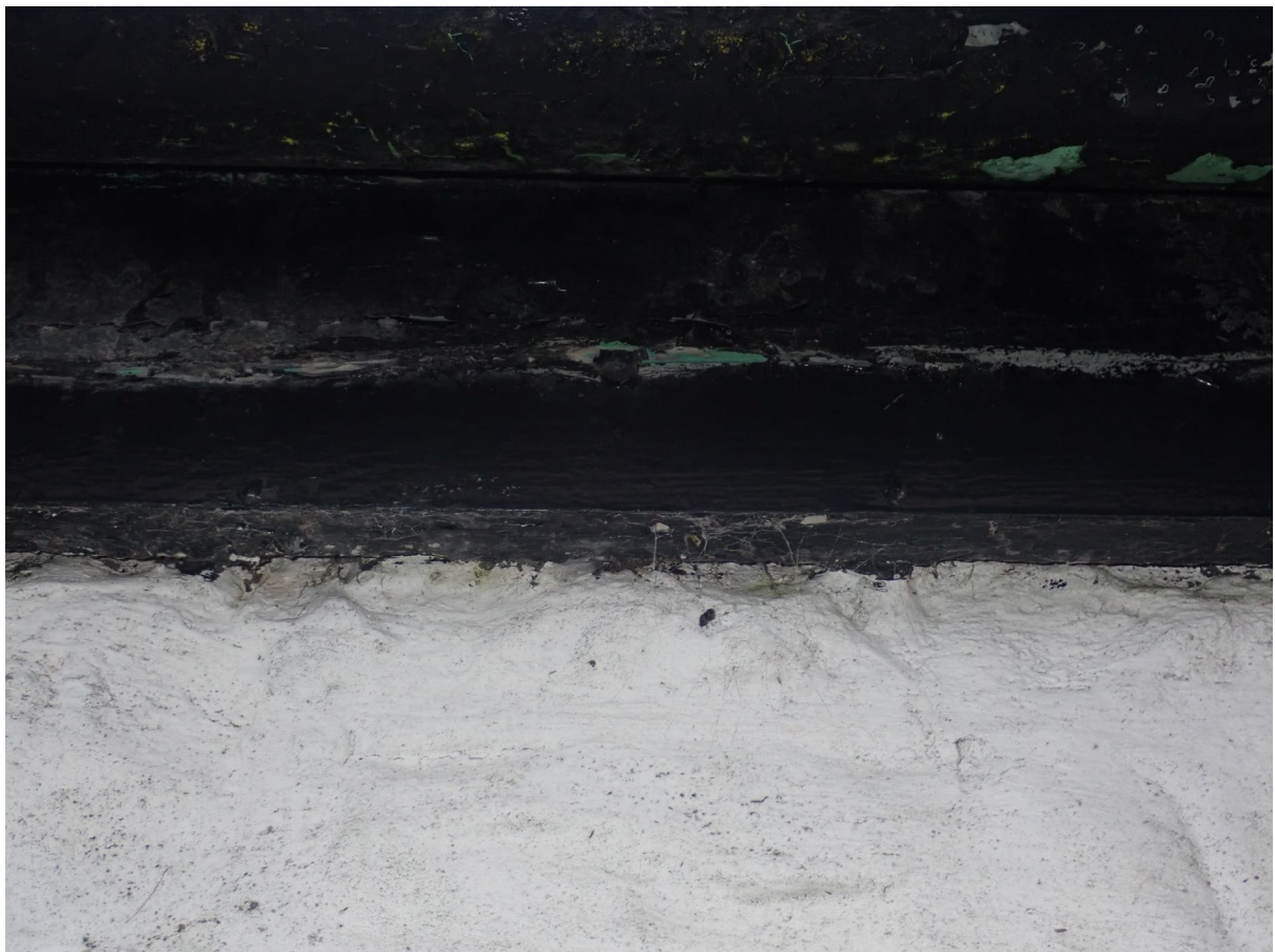
8 – Fascia boards where present are fitted tightly with no suitable gaps.
