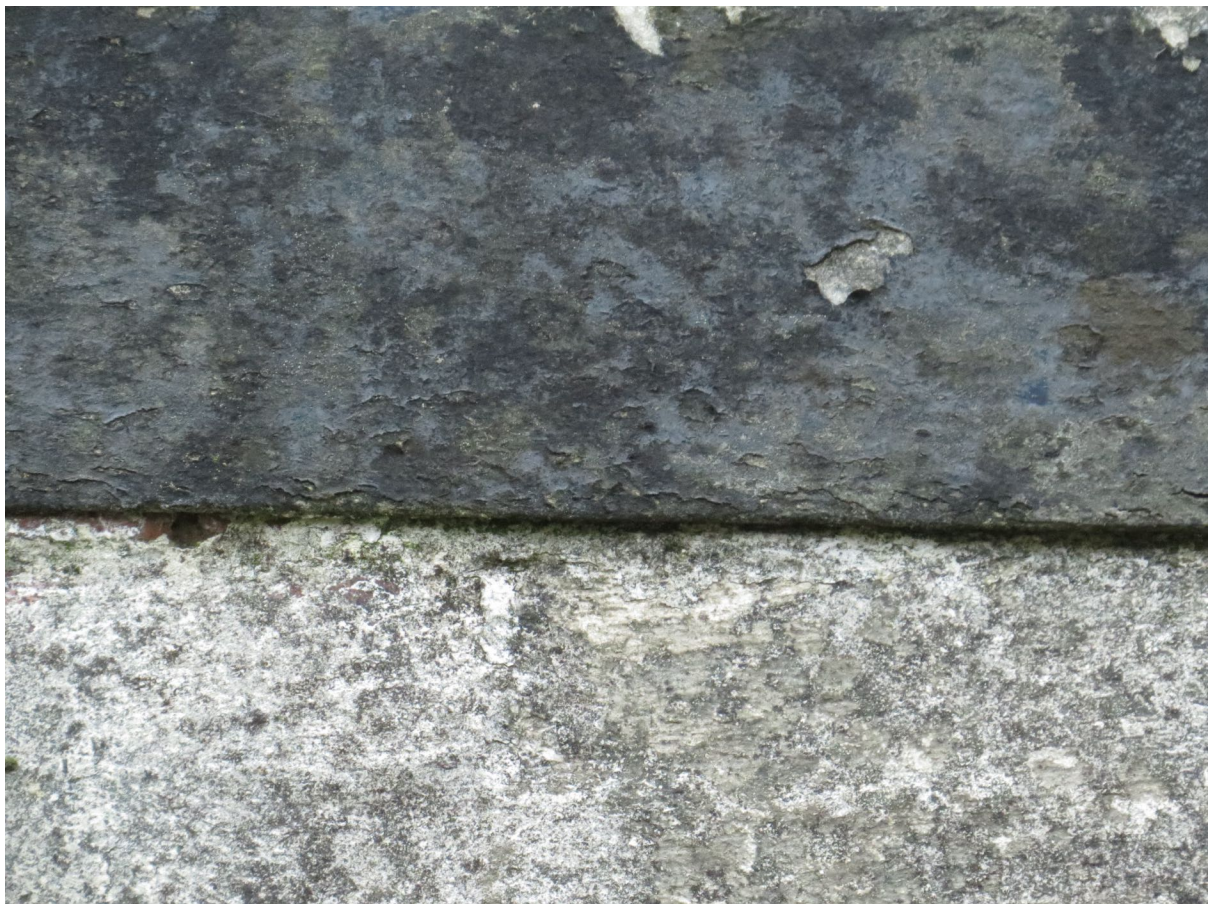
6 – Asbestos cement fascia are fitted tightly with no gaps.
