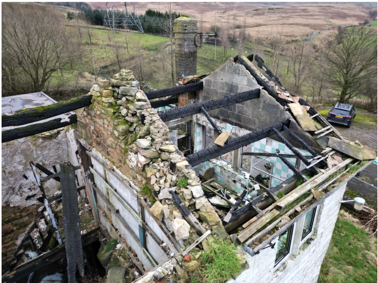
4 – Gaps in stonework and timbers at the top of the walls are open to the elements.
