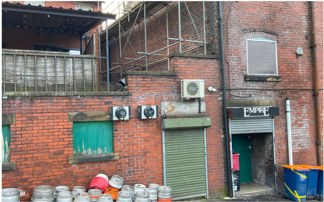
Typical elevation to King Street showing wall mounted plant and infilled windows
