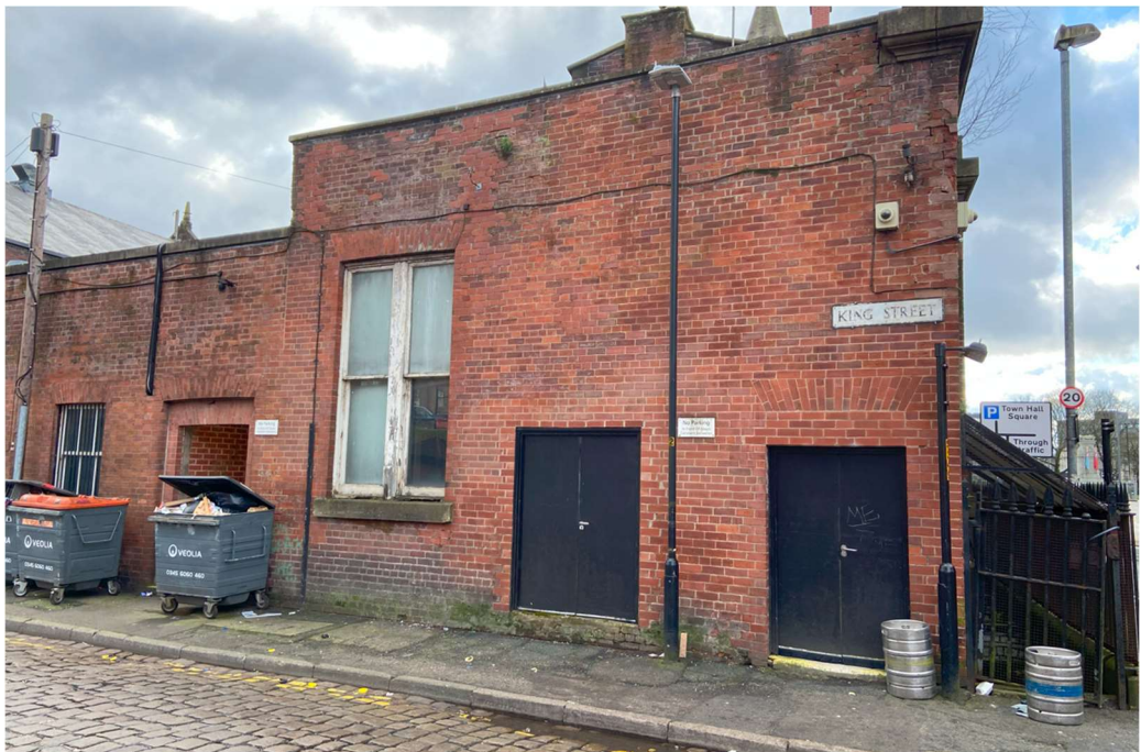
Gable to the rear of the Grade 2 listed Yates Wine Lodge showing infilled doors and new openings. Galvanised roof mounted flues are visible in the background
