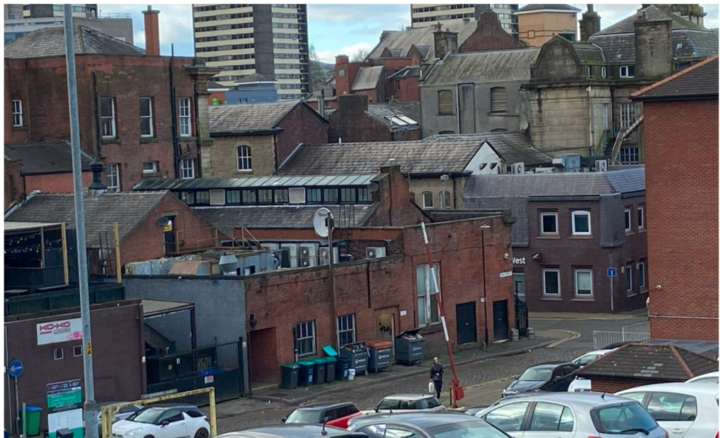
Roof mounted ventrilation kit and galvanised flues visible to roofs from Neson Street with the Job Centre visible to the right hand side
