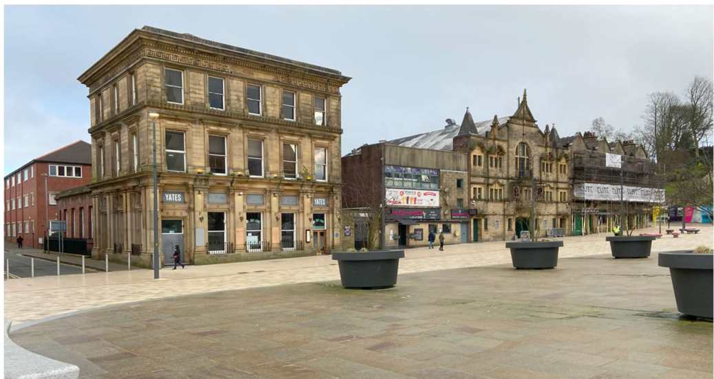
Elevation of buildings to east side of Packer Street with Job Centre gable to left side (the flue will not be visible from this vantage point)
