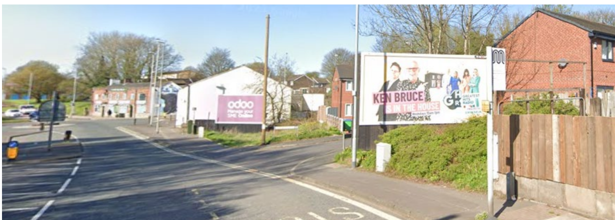
Figure 3 – April 2023 Google Street View of the Site
